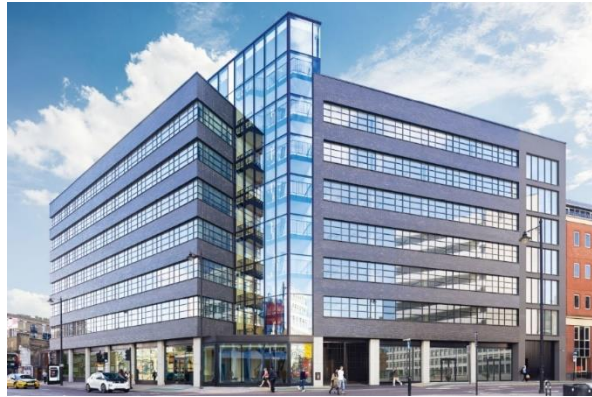
Figure 4 - Image of the extended and upgraded form of Arnold House showing continuity between new and existing structures. (© Allsop).
