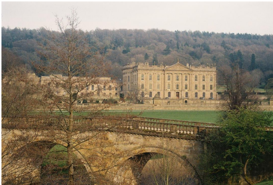
Figure 18 Chatsworth's west façade and bridge over the river Derwent
