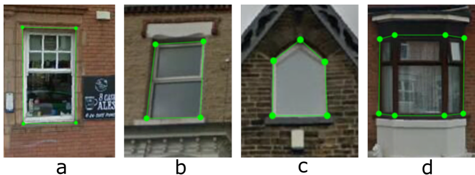
Figure 3.5: Examples of typical window annotations: including window frame but not including window sill and support beam as well as making a trade-off by slightly over-covering the window frame. a. a typical window with internal blind; b. a slightly inclined window; c. a window belonging to a loft; d. a typical bay window.
