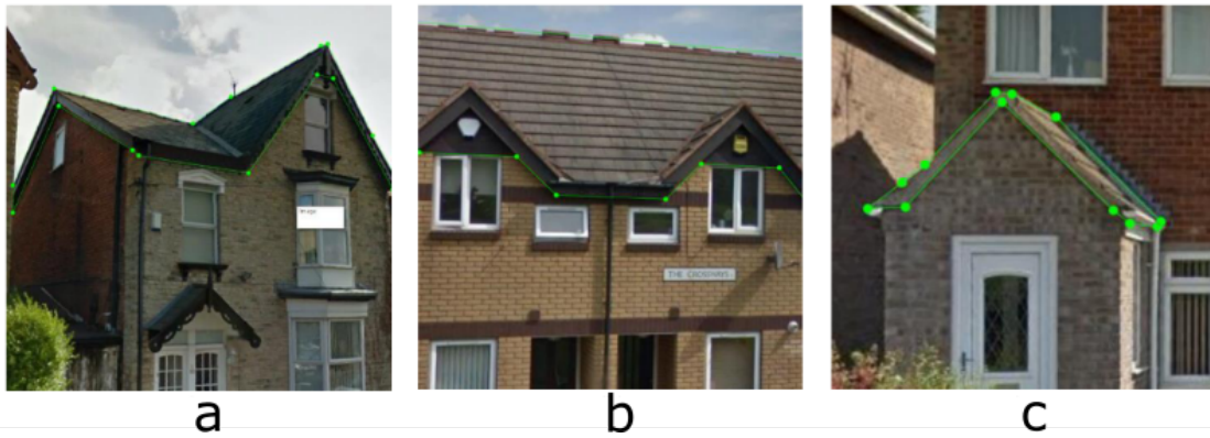
Figure 3.4: Examples of roof annotation. a. all parts belonging to a roof including eaves and rakes should be included; b. parts with materials that are different from the wall should be annotated as roof; c. ground floor roof structure should be labelled.
