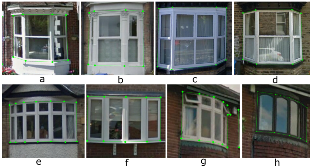
Figure 3.7: Examples of bay and bow window annotations. The top four examples show bay window annotations and the bottom four show bow window annotations. Bay window examples a, c, d should be put into standard window class and b should be in the alternative window class. Bow window examples e and f should be in the standard class and g and h should be in the alternative.
