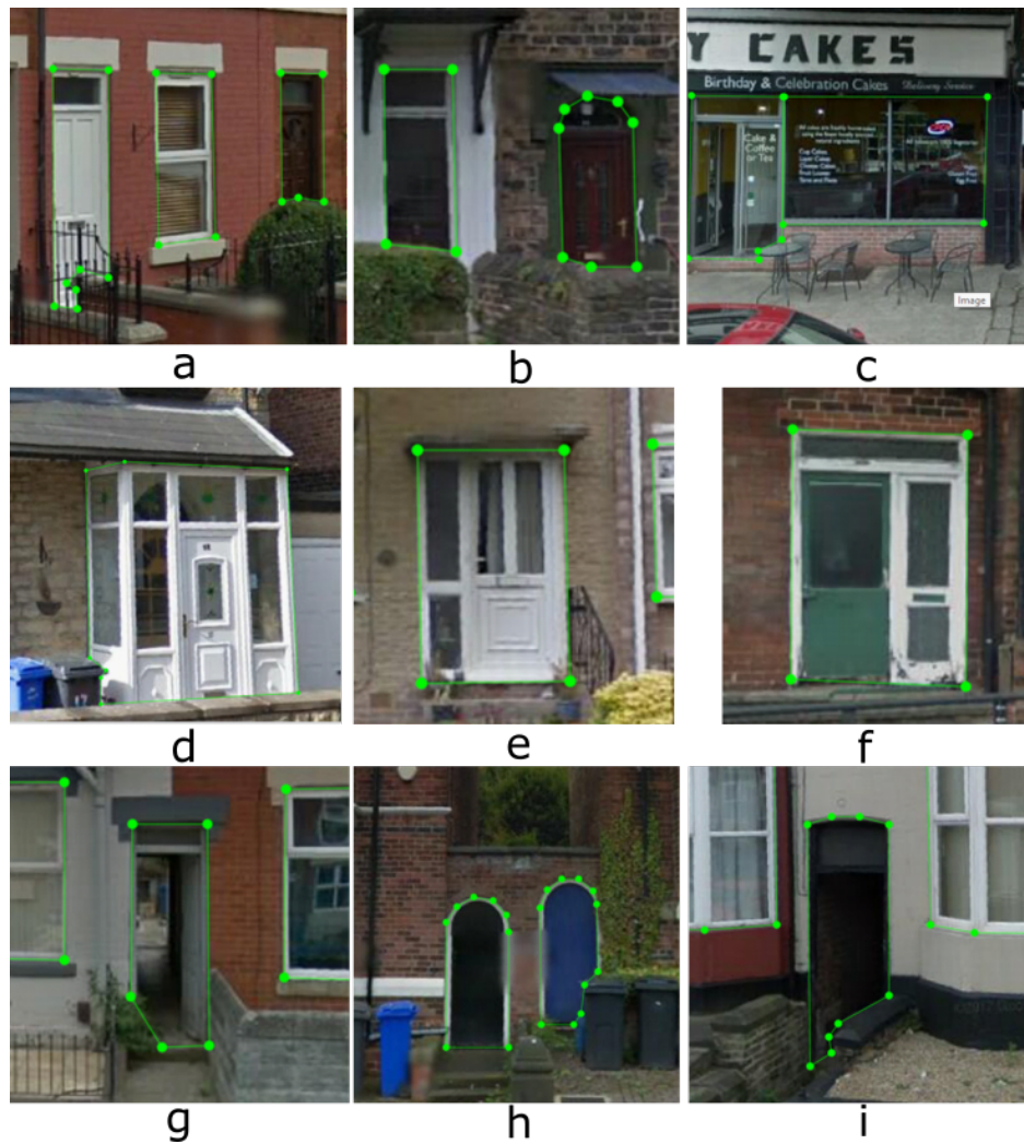
Figure 3.9: Alternative door annotation examples. Examples a,b and c show partially occluded, and opened door annotations. Examples d, e and f show annotation of extended-frame doors: all areas within the door frame should be labelled as the same door. Examples g, h and i show annotation of outer corridor doors.
