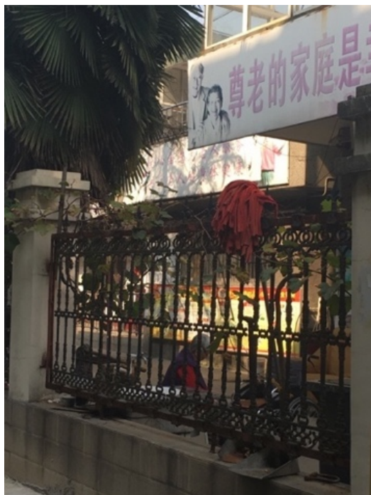
Figure 6: Exterior of Care Facility, Bengbu
