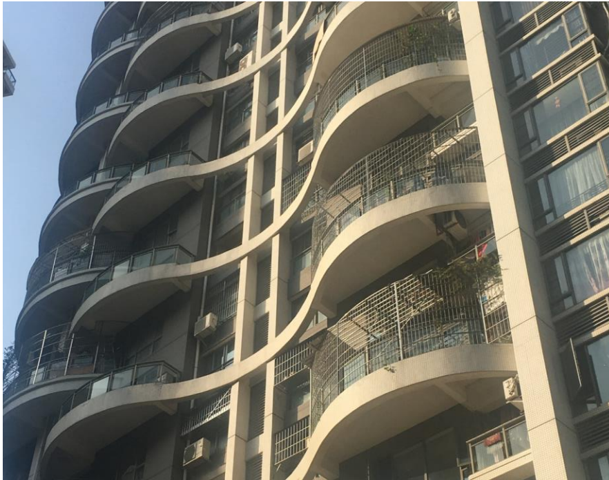
Figure 5: Installed iron grills on their balconies and windows
