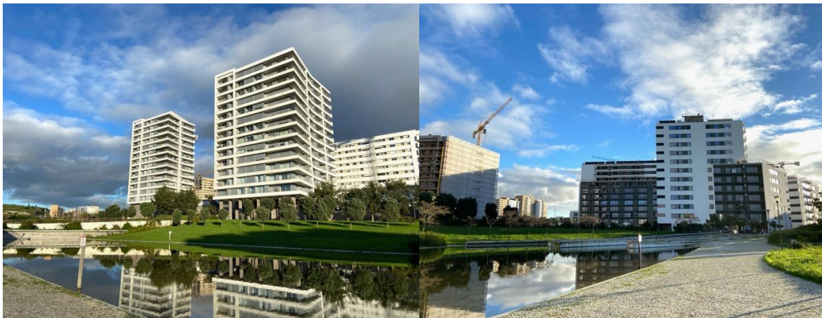
Figure 12: Two sections of Solyd's Altear project, completed (left) and under construction (right), in the outer Lisbon parish of Lumiar. Photos by author.
