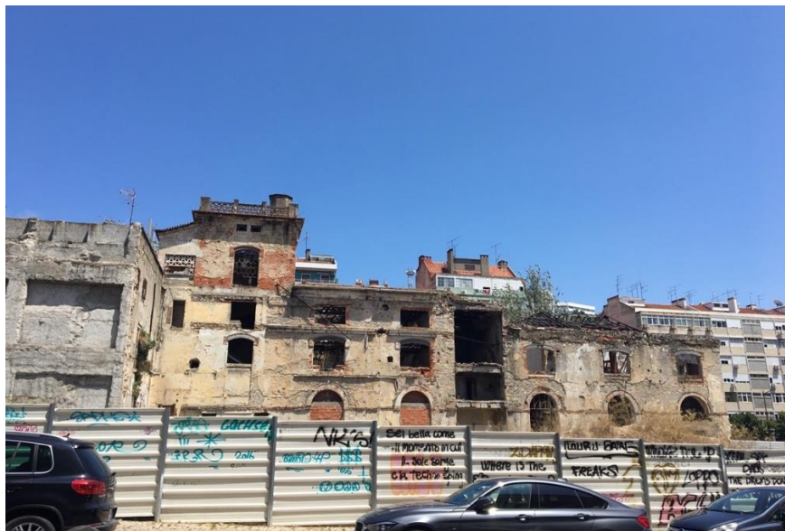
Figure 15: Part of the mostly demolished Portugália block in 2019, along the Avenida Almirante Reis. Photo by author.
