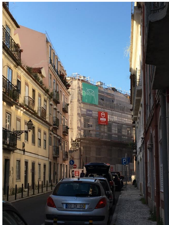
Figure 6: Rehabilitation in Lisbon's historic centre. Photo by author.
