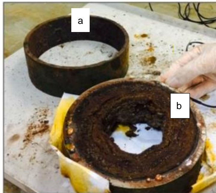
Figure 1. 5 - The cross section of a pipe (a) without scale deposited compared with a pipe (b) with scale[19].
