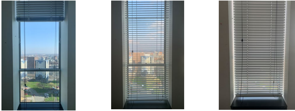
Figure 2-11: Horizontal blind: three opening conditions. In the left-hand image, the blind is raised completely to the top. In the middle image, the slats are in the horizontal position. The right-hand image shows the slats adjusted to the vertical position to completely block the view
