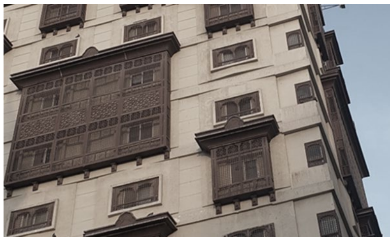
Figure 2-14: Example of mashrabiyya screening in the old city of Jeddah, Saudi Arabia; photograph © Wajdi Atwah, used with permission
