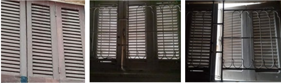
Figure 2-7: Photograph of types of external wood shutter window treatment in Libya. Left: the fixed slats are opened downwards, which is optimal for direct sunlight and privacy. Middle: this provides a very dark interior. Right: for ventilation and daylight, the panels of the screen can be rotated
