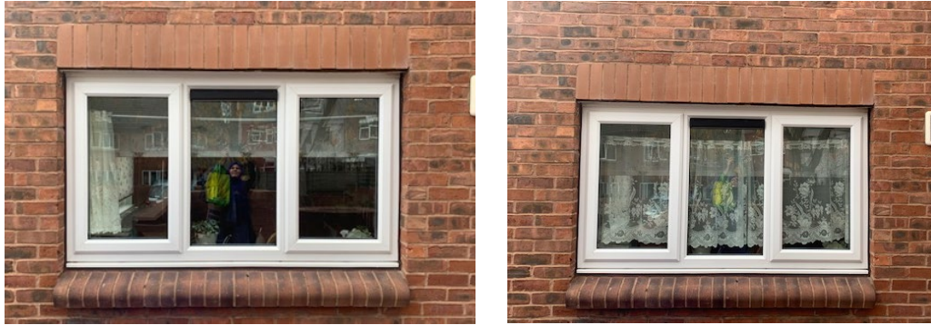
Figure 7-1 The effect of the reflection on the glass and the difference in luminance between outside and inside the house on visual privacy. The left image: the window without window treatments. The right image: the window covered by a curtain.
