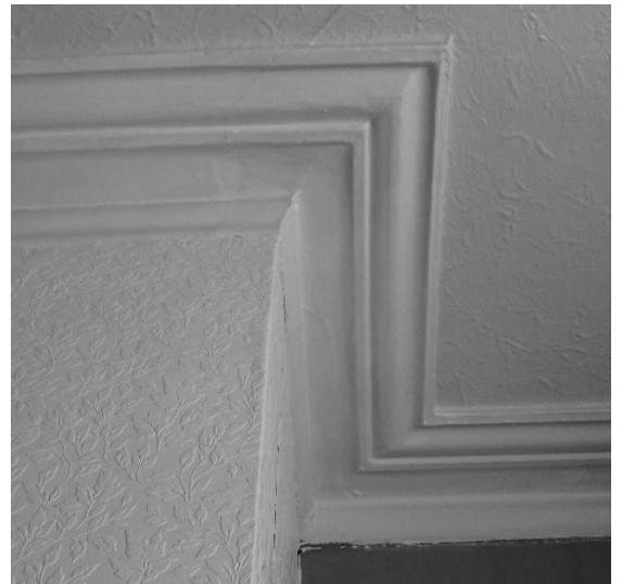
Figure 19 The original cornice in the living room.
