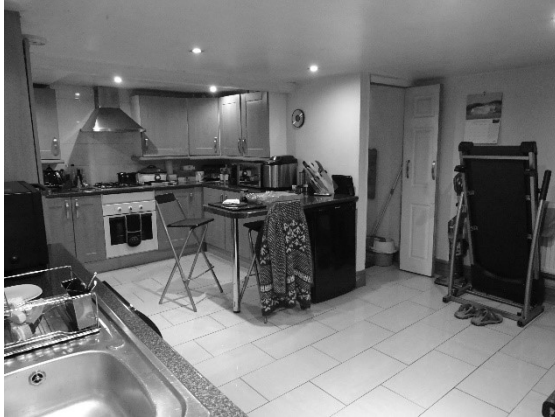
Figure 22 The entire basement area (including external WC) has been opened into one large space.
