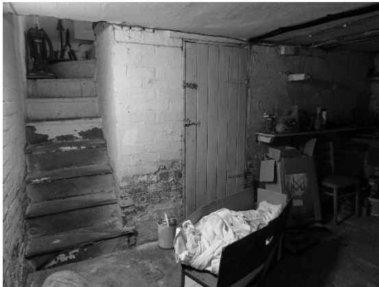
Figure 21 The largest of the three basement rooms.
