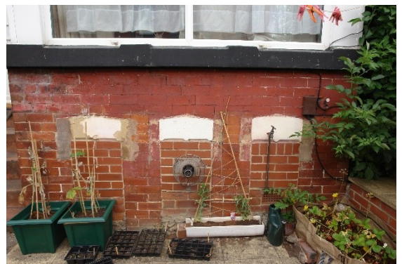
Figure 16 The three basement windows have been bricked up.
