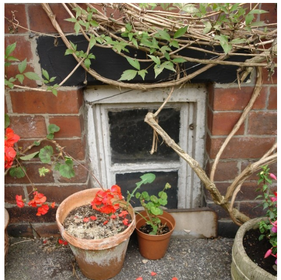
Figure 18 Part of the original basement window remains.
