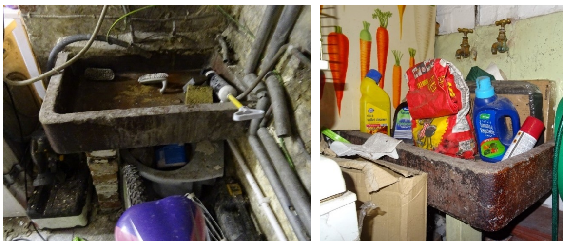
Figure 271 Salt-glazed wash cellar sinks.
