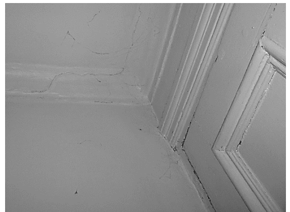
Figure 16 The living room cornice, architrave and panel door with heavy mouldings.
