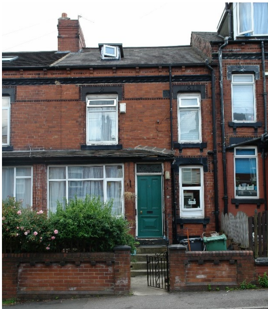
Figure 5 The house retains the essence of the original character.
