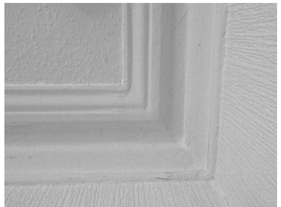
Figure 28 The living room cornice.
