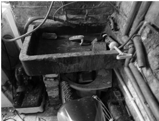
Figure 11 The original wash cellar sink.
