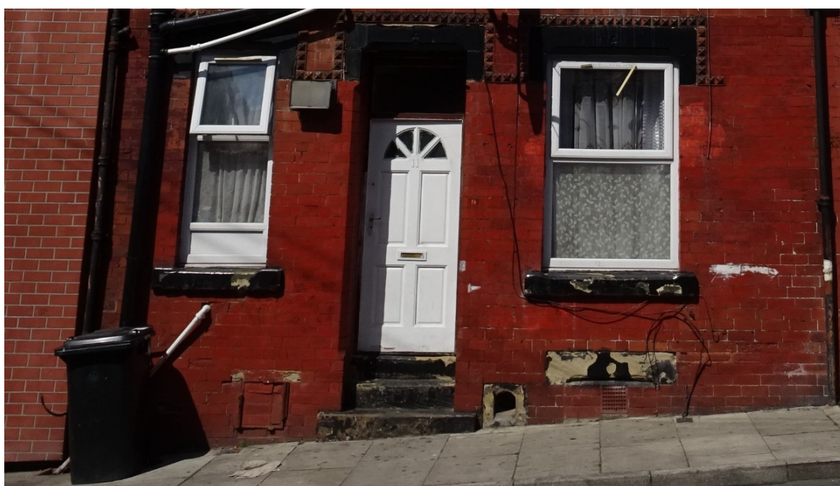
Figure 274 Type 2 street-lined house with entrance steps integral to the plan, a window at pavement level (now bricked up and with the lightwell filled and grate removed), a coal grate (now bricked up), and a boot-scraper next to the door (now badly damaged).
