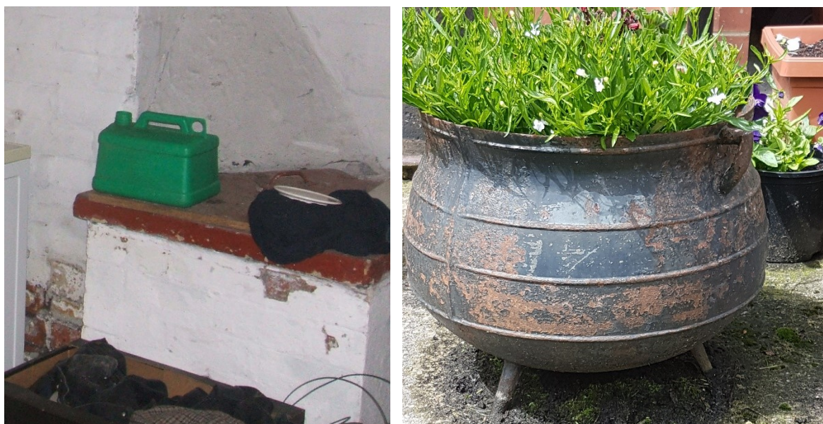
Figure 270 Set-pot housing - brick casing with a stone top and vented into the chimney stack (left); Set-pot inner 'copper' now used as a flowerpot (right, Childs 2019b).
