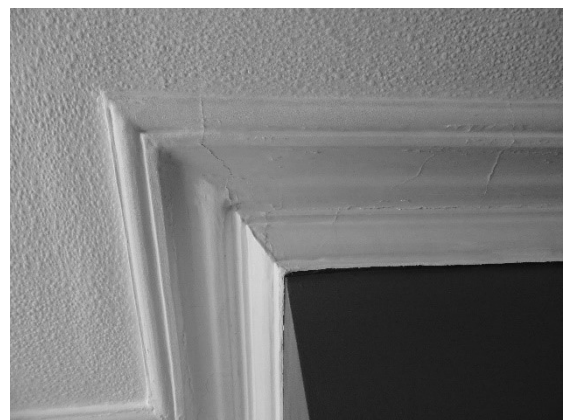
Figure 17 The cornice to the living.
