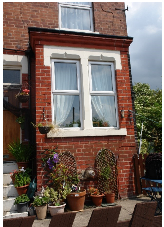
Figure 17 The square bay window includes a paired window with stone mullion and a decorative cornice detail at gutter level.
