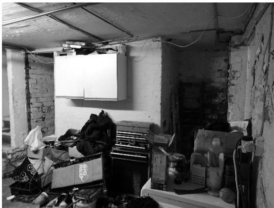
Figure 10 The largest of the basement rooms.
