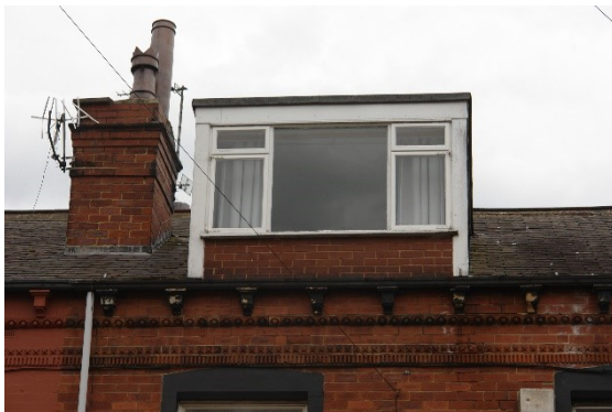
Figure 16 The roof has been modified with the addition of the dormer roof, but the original slate finish remains, as does one of the original chimney pots.
