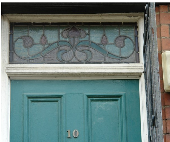
Figure 7 The original front door and stained glass fanlight. The fanlight is influenced by early 20 th century styles.
