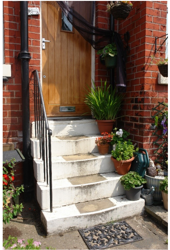
Figure 16 The original stone steps and balustrade remain in reasonable condition.
