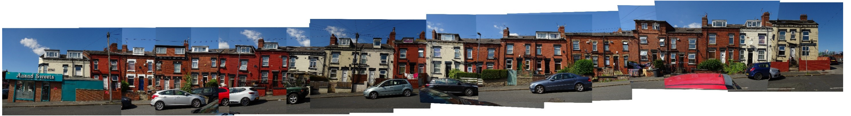
Figure 137 Ashton Street, North side.
