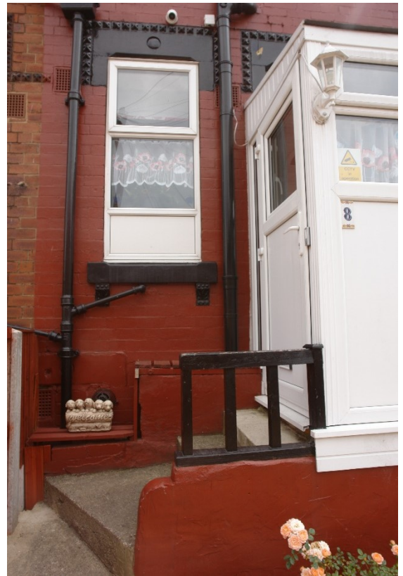
Figure 14 The entrance area to the house has been modified by replacement steps and a porch.
