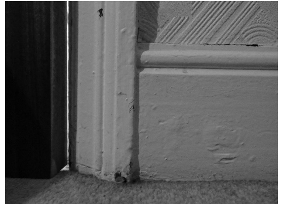
Figure 26 Original architrave (top); and skirting board (bottom).
