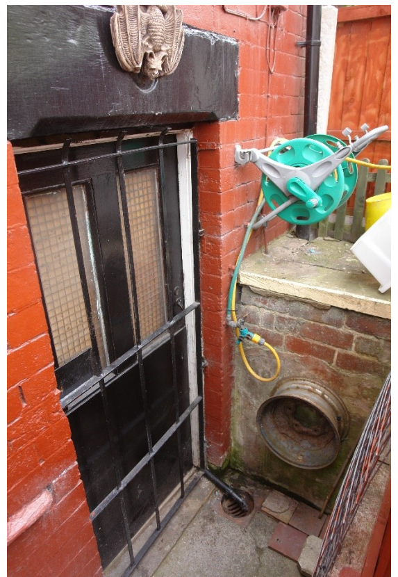
Figure 15 The original basement door remains in good condition.
