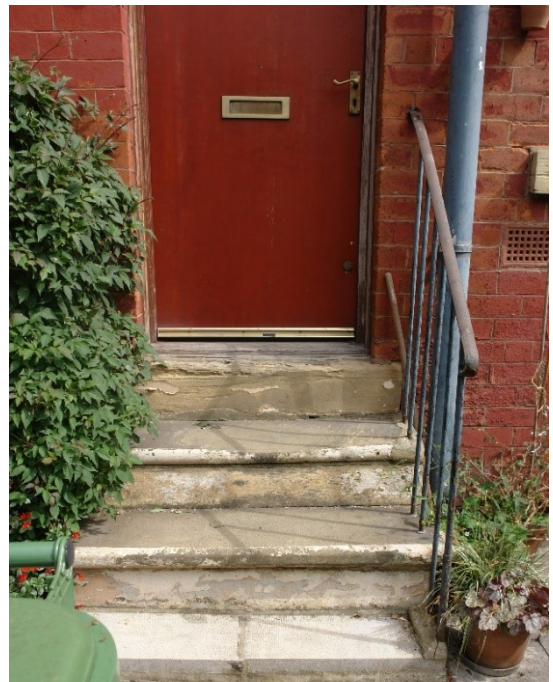
Figure 15 The original entrance steps and balustrade remain in reasonable condition.
