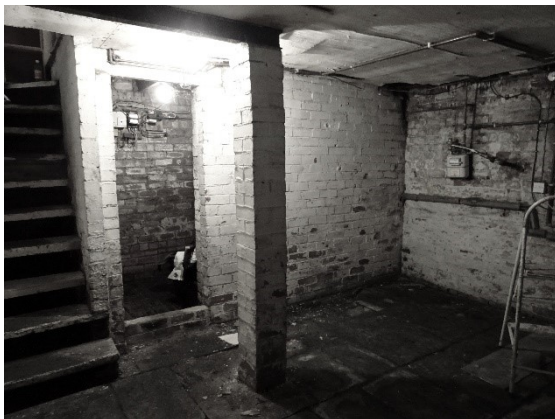
Figure 26 The column to the middle of the basement with the steel beam above, provided additional support to the house during wartime.
