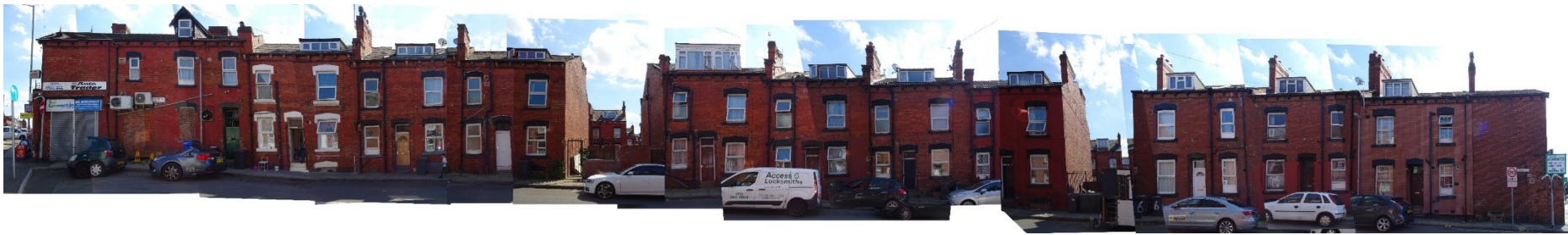
Figure 163 Lambton Street, South side.
