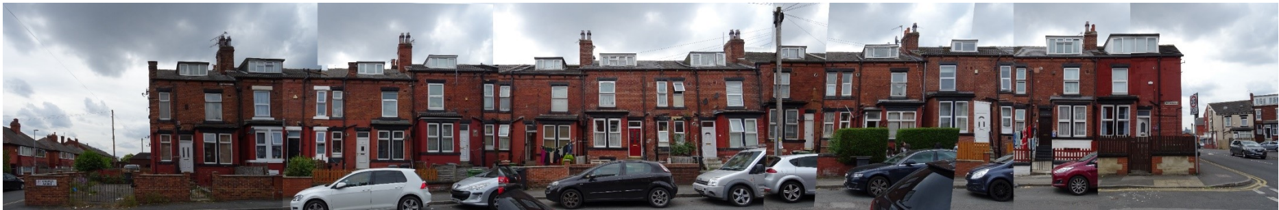
Figure 151 Cowper Avenue, West side.
