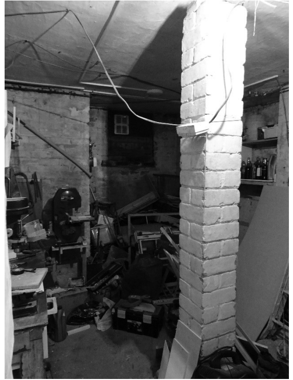
Figure 30 The window to the large basement room has been bricked up. The column gave additional strength to the house during war time.
