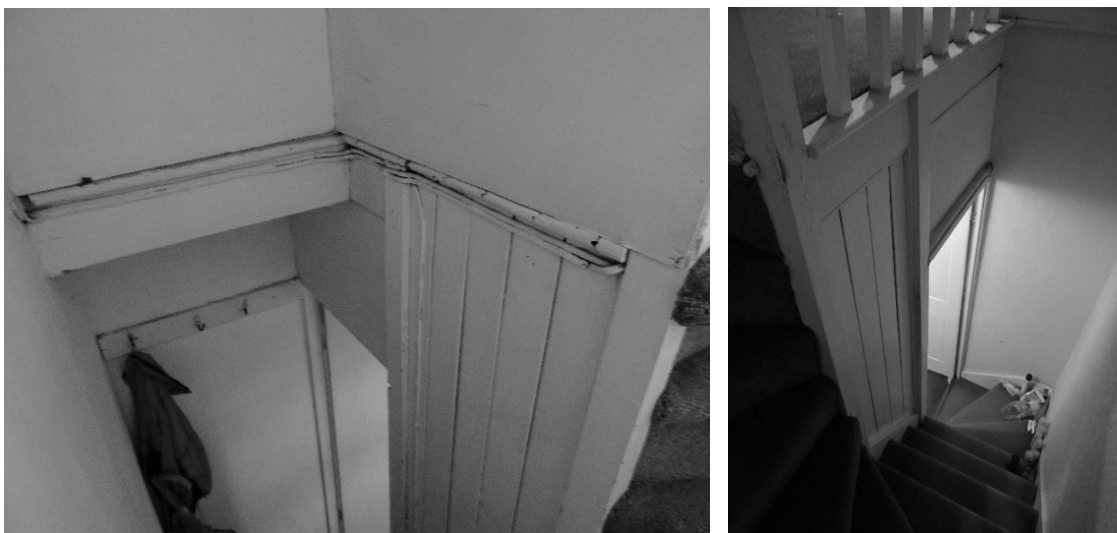
Figure 267 Most houses have full height panelling to the central staircase support. The floor edges are clearly visible, demonstrating a utilitarian approach to construction, and one which is innately honest about both the nature of construction and the need to maximise every inch of available space.
