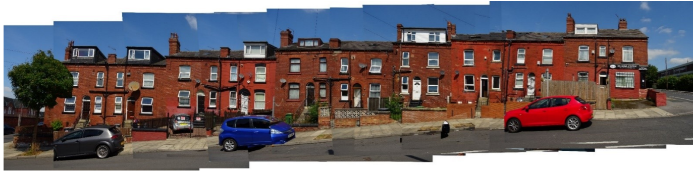
Figure 148 Conway Mount, North side.
