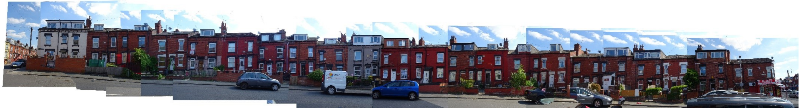
Figure 138 Ashton Street, South side.
