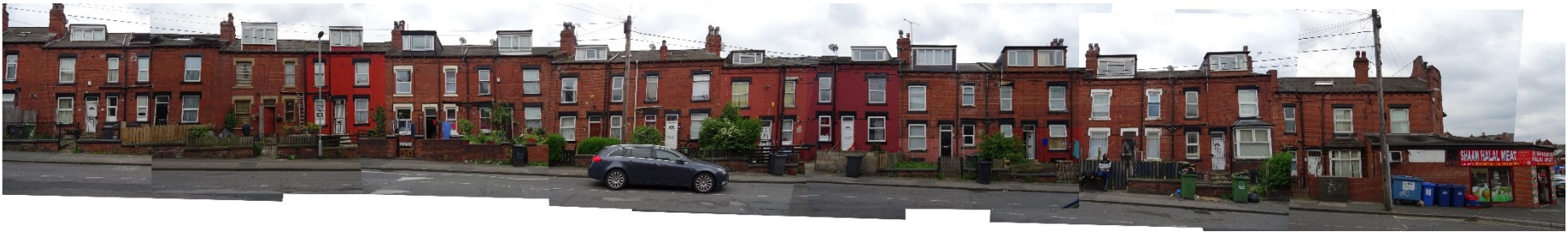
Figure 135 Ashton Grove, South side.
