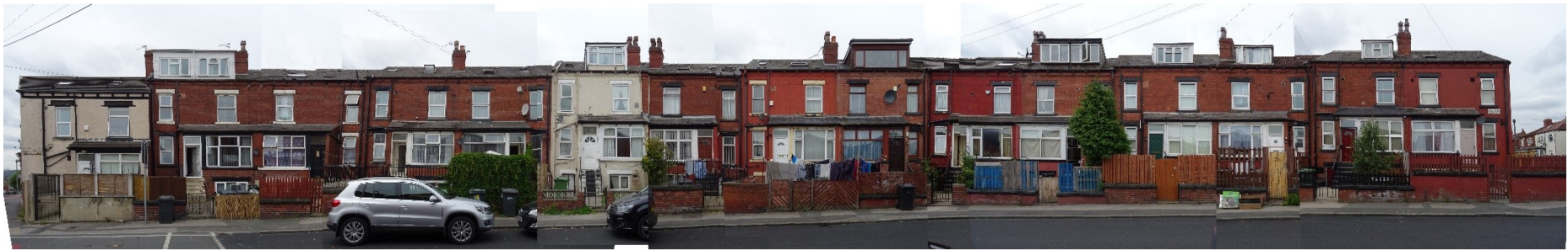
Figure 156 Darfield Road, West side.
