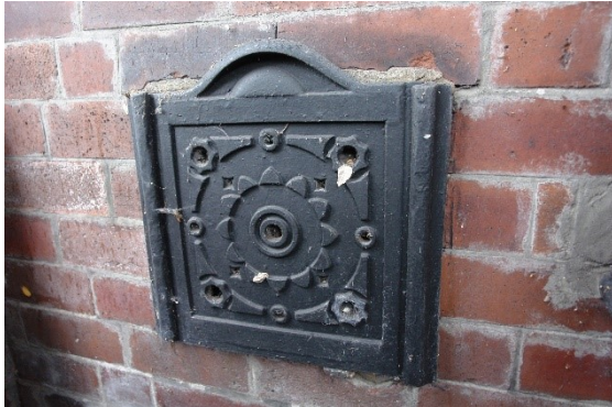
Figure 20 The coal grate is in excellent condition.
