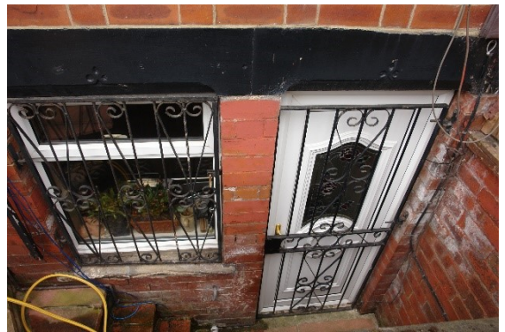
Figure 16 The basement entrance area.
