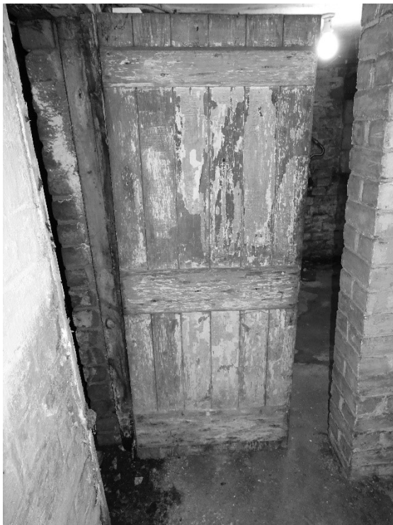
Figure 16 The original coal cellar door.
