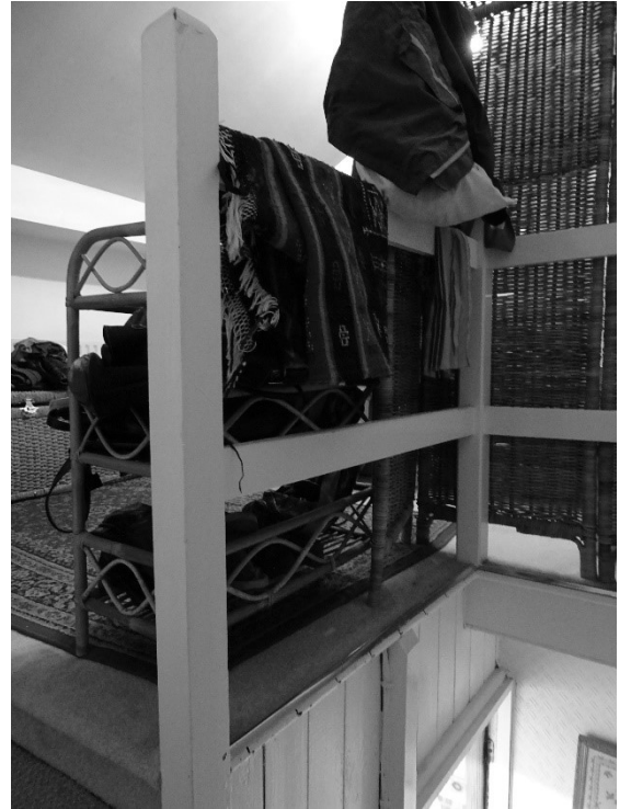
Figure 25 The original staircase construction and newel posts in the attic.
