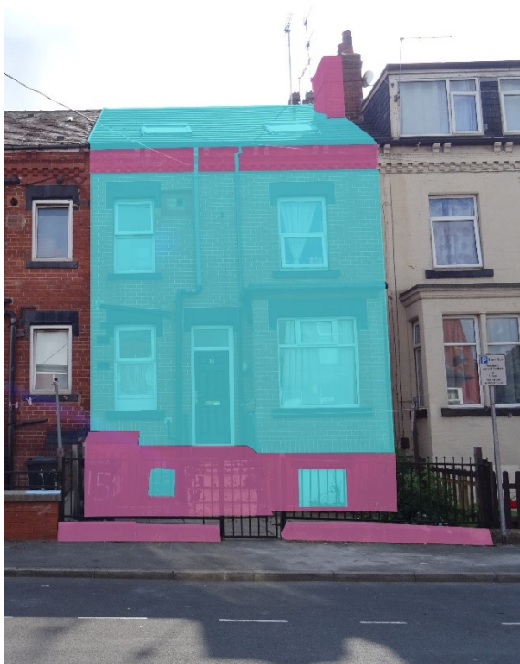
Figure 48 Bexley Place — Low retention of original fabric.
