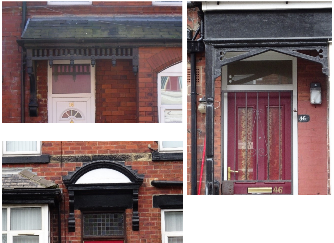
Figure 16 Timber porches and canopies.
