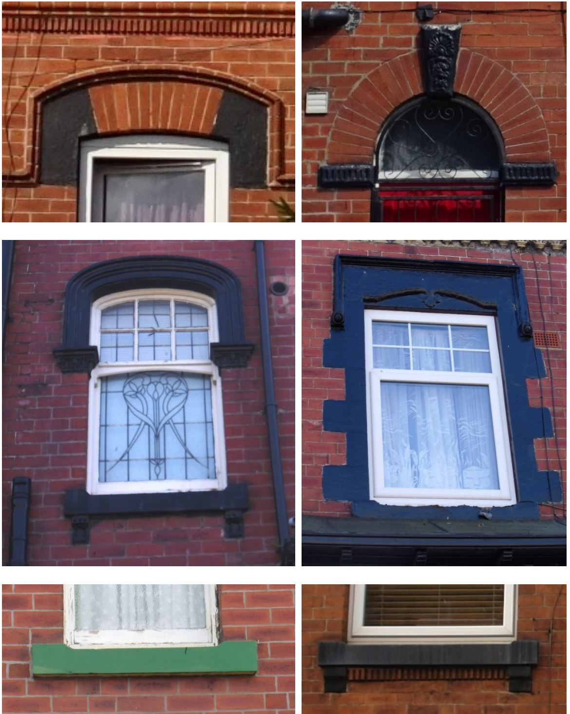
Figure 13 Stone and brick combinations used in arched lintels (window, top left; door, top right); curved stone lintel supported off corbels (middle left); stone lintel with reveal quoins (middle right); plain sill (bottom left) and sill supported off corbels with decorative brick between (bottom right).
