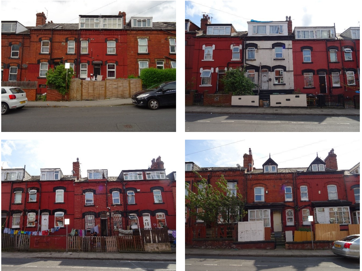
Figure 36 The modification of boundary walls has radically altered the uniformity of the streetscape in ways that seemingly reflect individual preferences and eclecticism; a rebuilt wall and tall fence (top left); rebuilt wall, rendered wall and railings in lieu of the wall (top right); ad-hoc mixture of replacement rendered walls and palisade fencing (bottom left); fencing (ageing, makeshift and full height) on and behind the original walls (bottom right).
