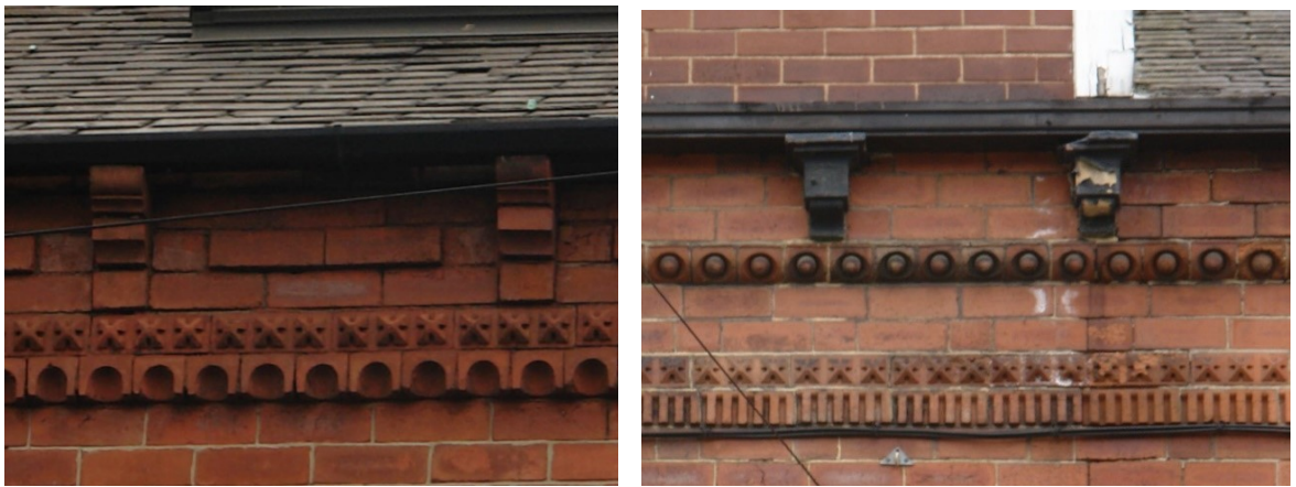
Figure 11 Brick gutter corbels (left); and stone corbels (right) support square timber gutters.
