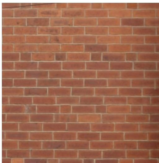
Figure 8 The brick bond is the same across the entire neighbourhood, regardless of construction date, and comprises five rows of stretchers and one row of alternate headers and stretchers. Lime mortar joints are narrow, at approximately 3/16" to 3/8" (4.5-10mm) thick.
