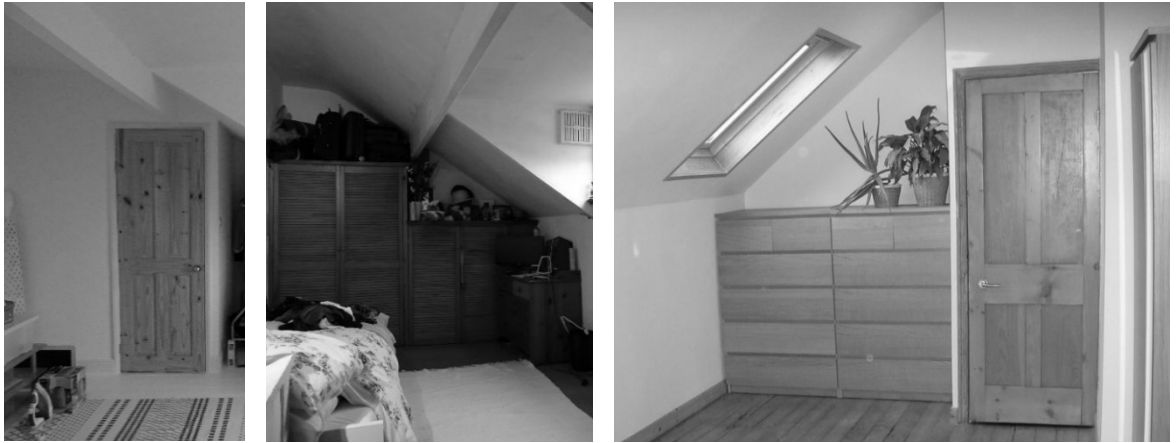
Figure 10 Purlins are positioned at variable heights throughout the neighbourhood: immediately below the flat ceiling (left); at high level, mid-way along the sloping ceiling (centre); and at the height of the dwarf wall and concealed within (right).
