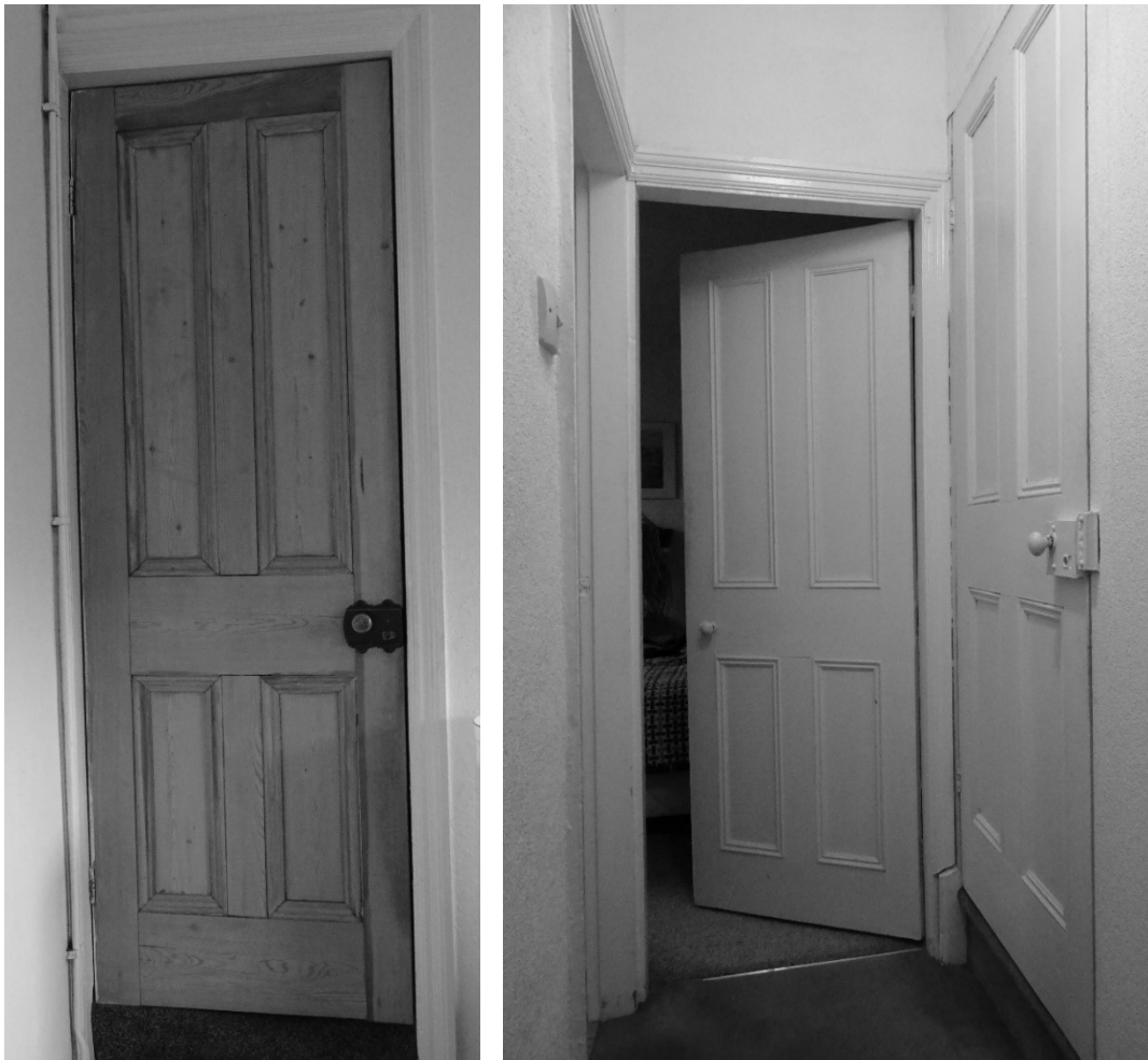
Figure 19 Four-panel doors complete with planted mouldings and original ironmongery.
