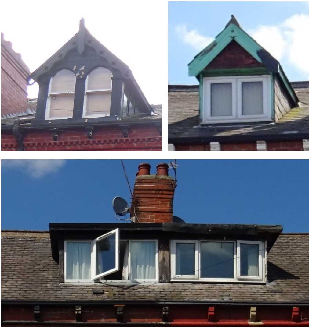
Figure 15 In Character Area 1, gable dormers had decorative bargeboards, a gable post and glazed cheeks (top left) while in Character Area 4 houses, bargeboards were plainer and cheeks had a slate finish (top right). A notable exception to the centrally positione
