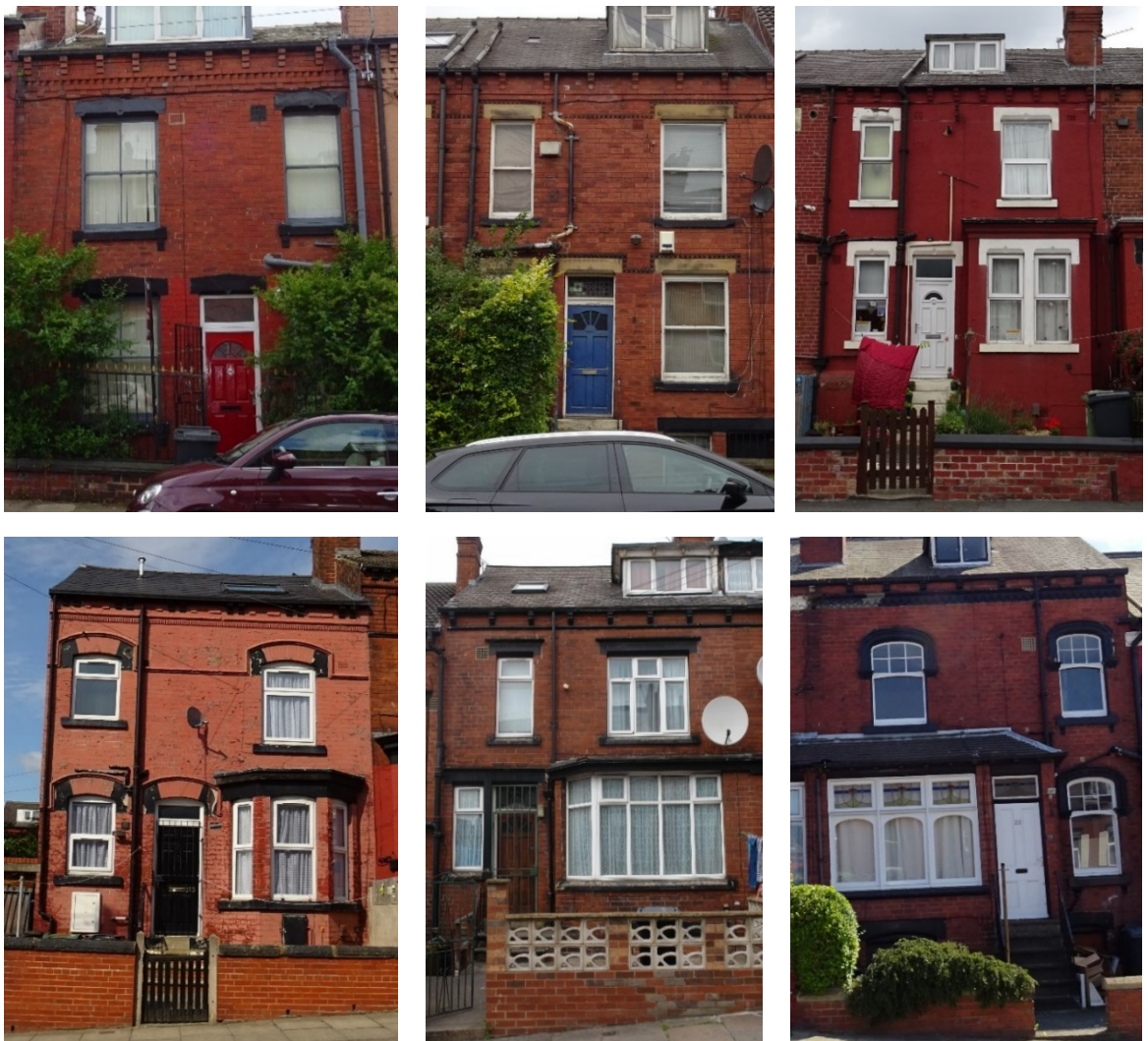
Figure 14 Sliding sash windows with glazing bars (top left); Sliding sash windows with horns (top middle); Square bay window with paired sashes and stone mullion (top right); Semi-hexagonal bay with three sashes (bottom left); Splayed bay with casement window (bottom middle); Bay with pitched roof extended over the porch. Casement window to bay, and small top sashes with curved transom and glazing bars (bottom right).
