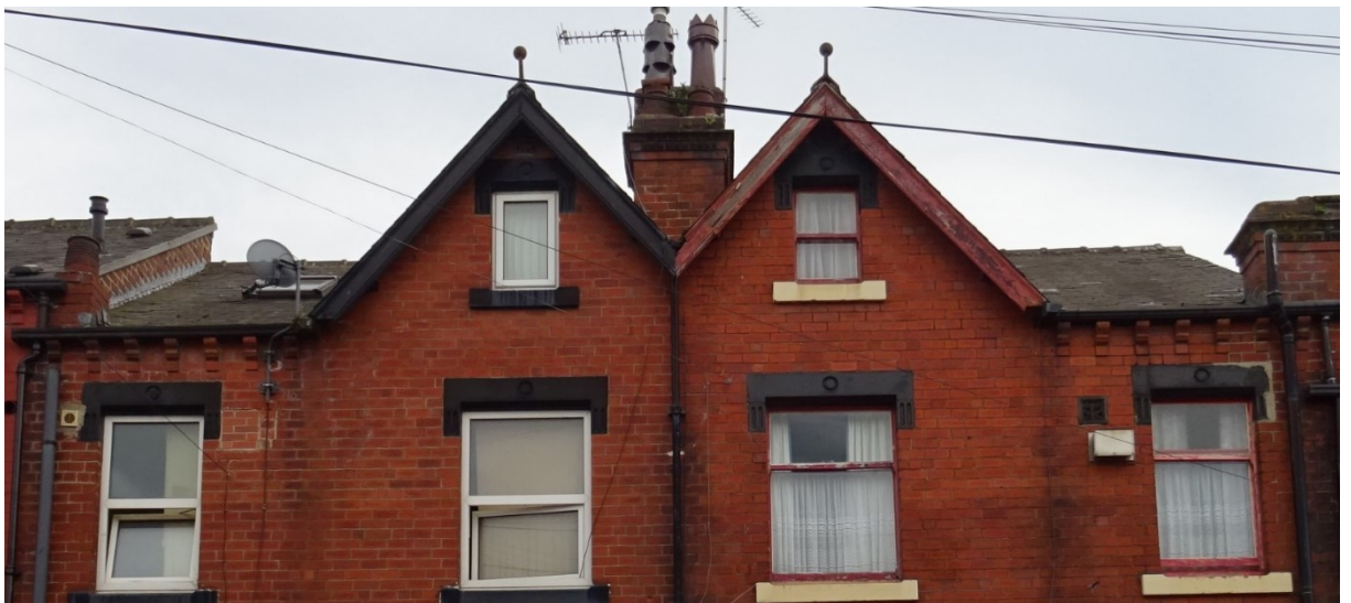
Figure 9 In the houses without attic rooms, the roof pitch commences at first-floor ceiling level (top) whereas in those with attic rooms, extension of the wall above the first-floor ceiling level before the roof pitch commences, gives additional headroom in the attic (middle). A minority of houses have cross gables (bottom).
