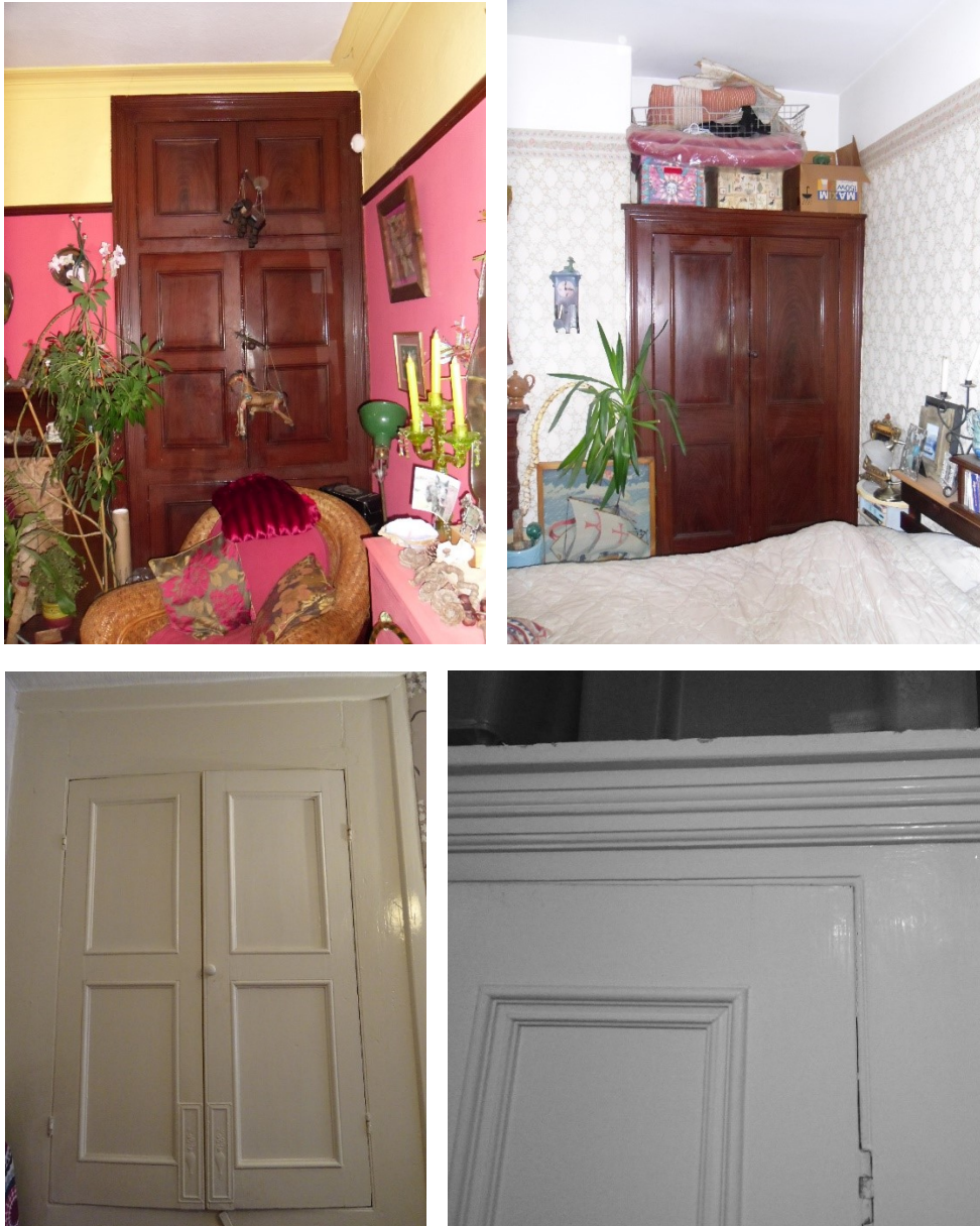
Figure 24 Full height built-in cupboard to the rear living-kitchen alcove, finished in a faux wood grain glaze (top left); the matching bedroom storage in the room above, with a reduced height and decorative cornice to the top (top right); full height living-kitchen cupboard to a rear alcove, now painted white but with decorative fingerplates still visible (bottom left); detail of a built-in wardrobe to the front alcove, showing the design of the planted mouldings, architrave and cornice (bottom right).
