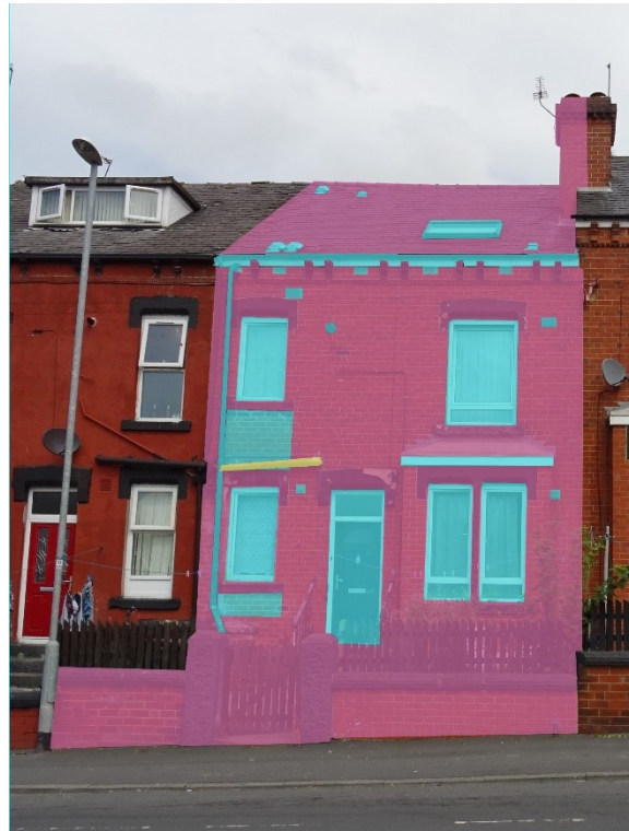
Figure 49 Bayswater Road — Medium retention of original fabric.
