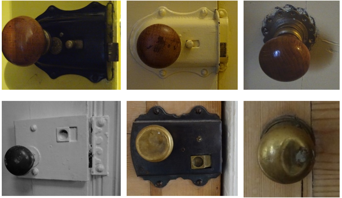
Figure 20 Surface mounted rim sash locks and handles have a metal case with a painted finish, a brass metal locking mechanism and a rose (to the other side). Handles are either brass or polished wood.
