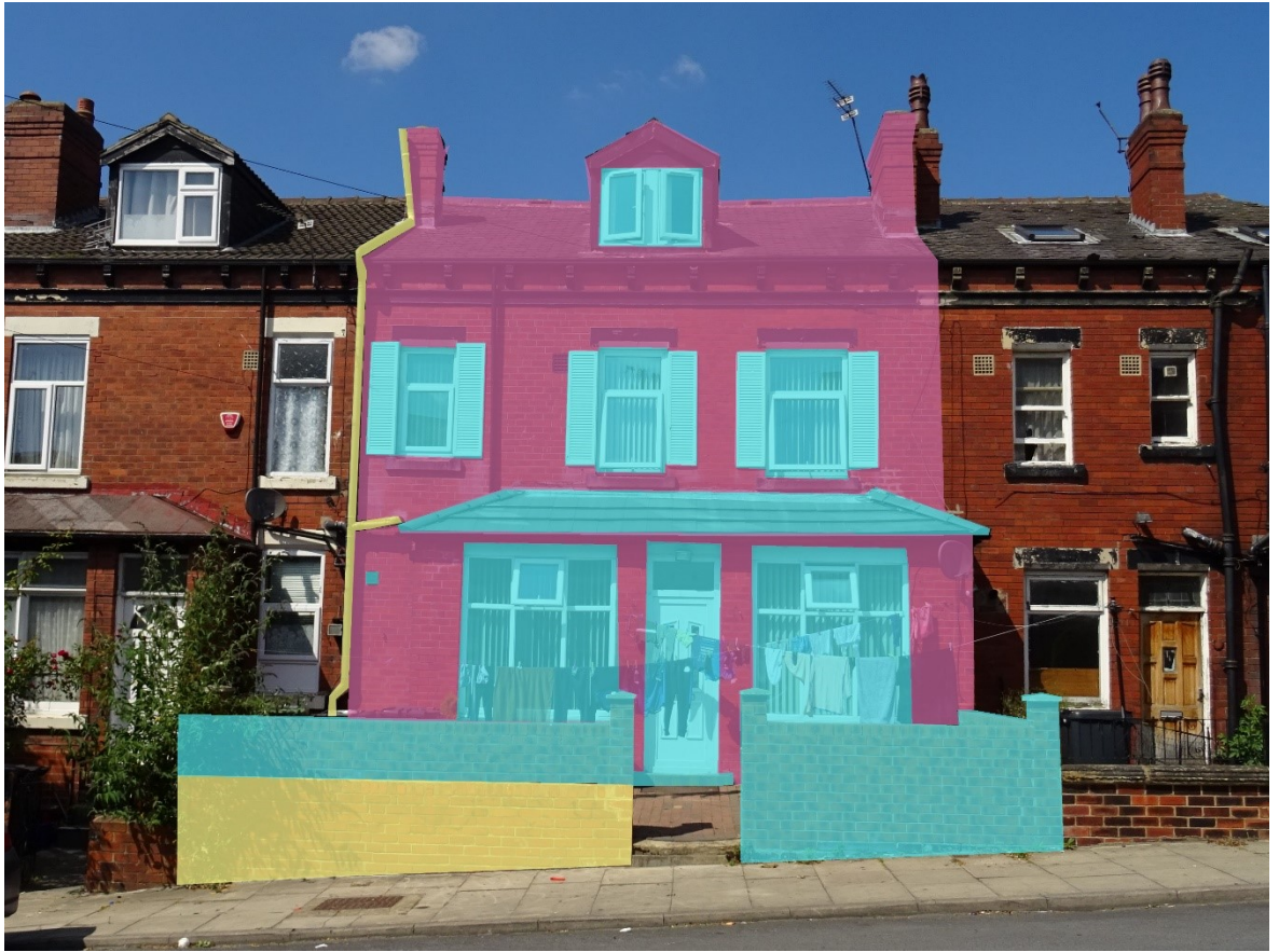
Figure 58 Luxor Road — Low retention of original fabric.
