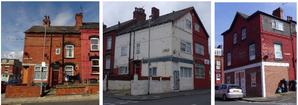
Figure 41 Little regard has been paid to the character or architectural language of the shop-houses converted to domestic use, with some being so poorly designed that they blight the streetscape.
