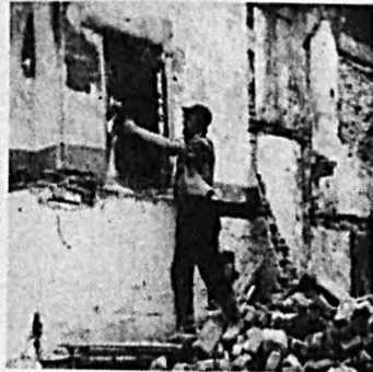
(RIGHT) Fig. 3—A closer view of the waiting room. The old grate you see being pulled out, I now have at home. Couldn't resist...
