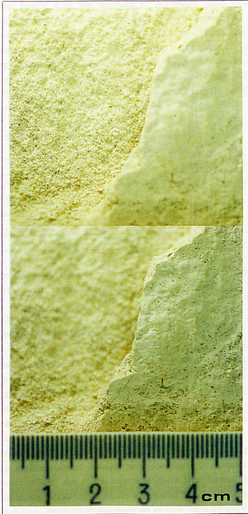
Plate 4.5: Photograph indicating different textures of the surface layer and the underlying material
