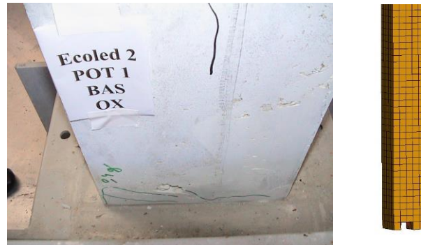
Figure 4.13 (On the left) concrete cracking and spalling in the base of the column observed in the experiment, (on the right) concrete erosion resembling cracking/spalling in LS-DYNA simulation
