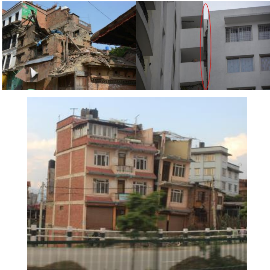
Figure 2.2 Collapse of buildings due to pounding in Bhaktapur during Gorkha earthquake in 2015 (Wijeyewickrema et al., 2015)
