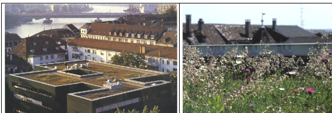
Figure 1.3. The green roof at Rossetti Research Building-Basel Hospital, Basel (Photos by Stephan Brenneisen; pictures from Earth pledge, 2005).
