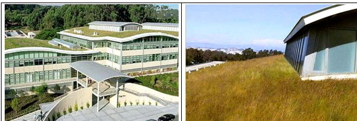
Figure 1.8. The green roof at the GAP headquarters, 901 Cherry (Pictures from greenroof.com).
