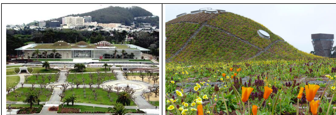
Figure 1.7. The green roof at the California Academy of Sciences (Pictures from greenroof.com and calacademy.org).
