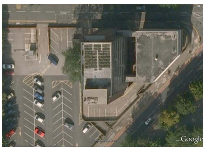
Figure 4.1. The experimental site (Source from: Google Earth).
