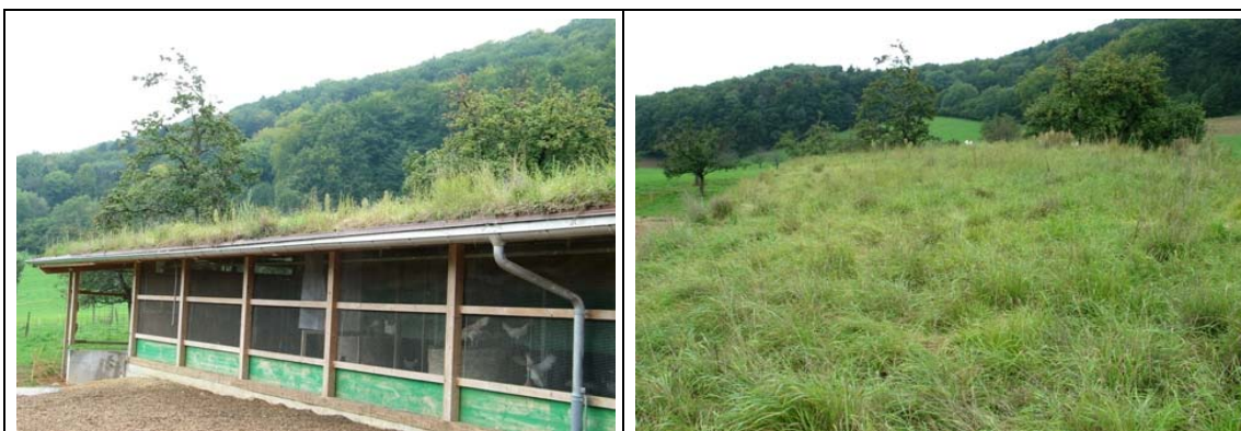
Figure 1.1. The green roof at Chicken barn, Asphof, Rothenfluh, blending the planting with the surrounding landscape (Photos by author taken on Sep 2005).
