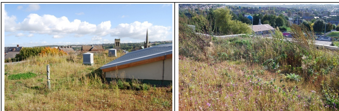
Figure 1.5. The green roof on Sharrow Primary School; spontaneous plants and annual meadow (Photos by author taken on Oct 2008).
