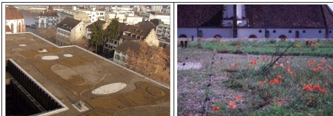
Figure 1.2. The green roof at the Klinikum 2 of the Cantonal hospital of Basel with substrate stimulating river terrace conditions (left: photo by Stephan Brenneisen, picture from Brenneisen 2006; right: picture from greenroofs.com).
