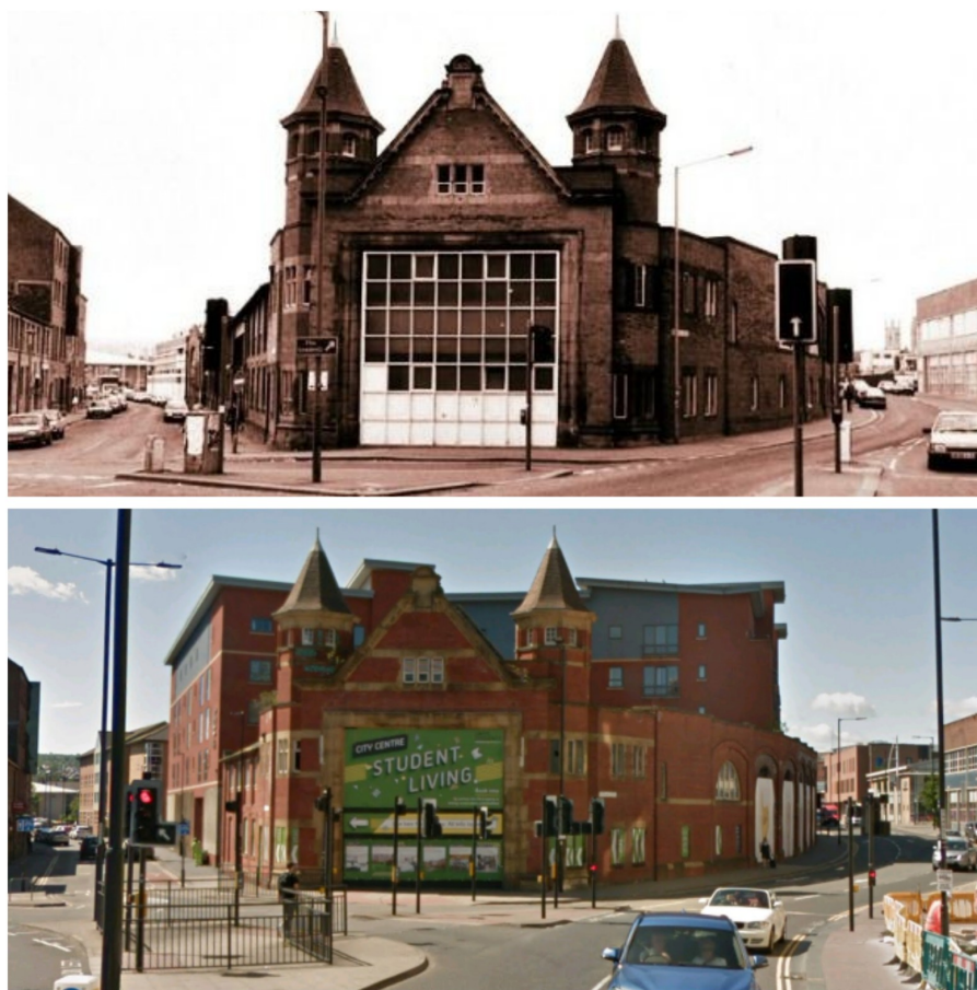
Figure 5.32: The Leadmill Tram Depot 1985 and 2019. Cultural Industries Quarter
