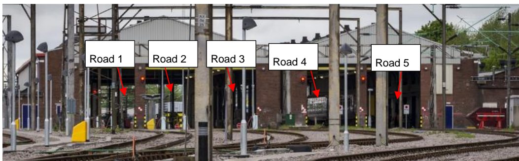
Figure 3.1 Main Shed of Allerton Railway depot, Liverpool, (Roads 1-5) (RTM, 2016)
