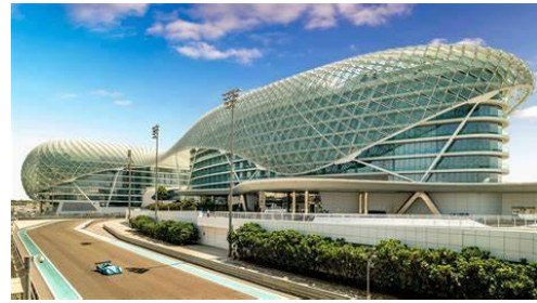
Source: https://visitabudhabi.ae/en/where-to-go/islands/yas-island Figure 6.12 The roof of Yas Island of Abu Dhabi
