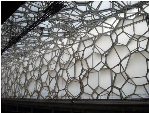
Source: https://www.arup.com/projects/chinese-national-aquatics-center Figure 6.13 The spatial structure of Water Cube
