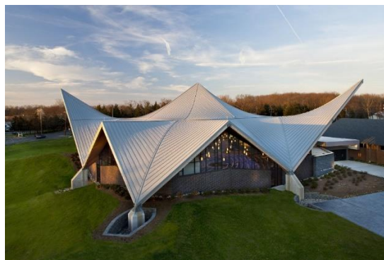
Source: https://www.metalconstruction.org/index.php/case-studies/St-Aloysius-Church-Jackson-NJ?case%5Bproduct%5D=1993 Figure 6.6 Hyperbolic paraboloid construction
