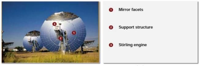
Figure 2-5: The PDS main components [49].
