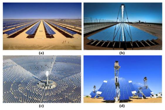
Figure 2-2: Main CSP technologies: (a) PTC; (b) LFR; (c) SPT; (d) PDS [42].
