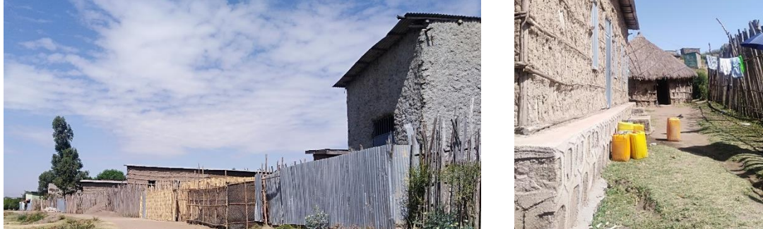
Fig. 24. Worker's housing built on farmland in Dato sub-city (by author in Jan 2019)
