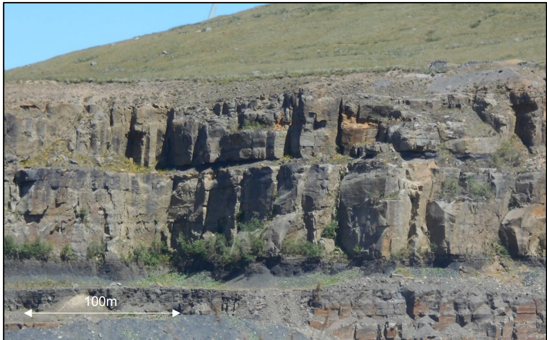
Figure C5: View of orthogonally jointed sandstone beds at Scout Moor Quarry, Ramsbottom, Lancashire
