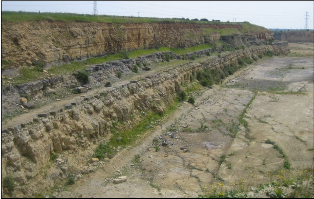
Figure 4.15: Tension cracking due to quarry floor heave at a 30 m deep quarry excavation in the Lincolnshire Limestone
