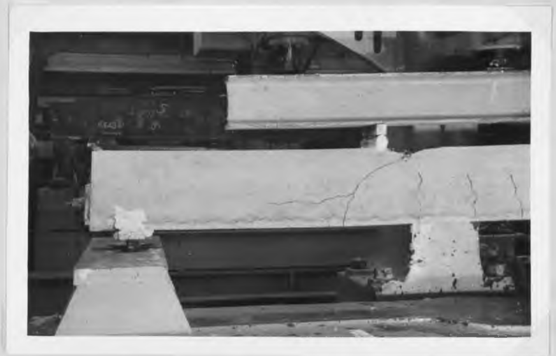
Plate 4 Cracking at the level of the reinforcement following the formation of the inclined crack
