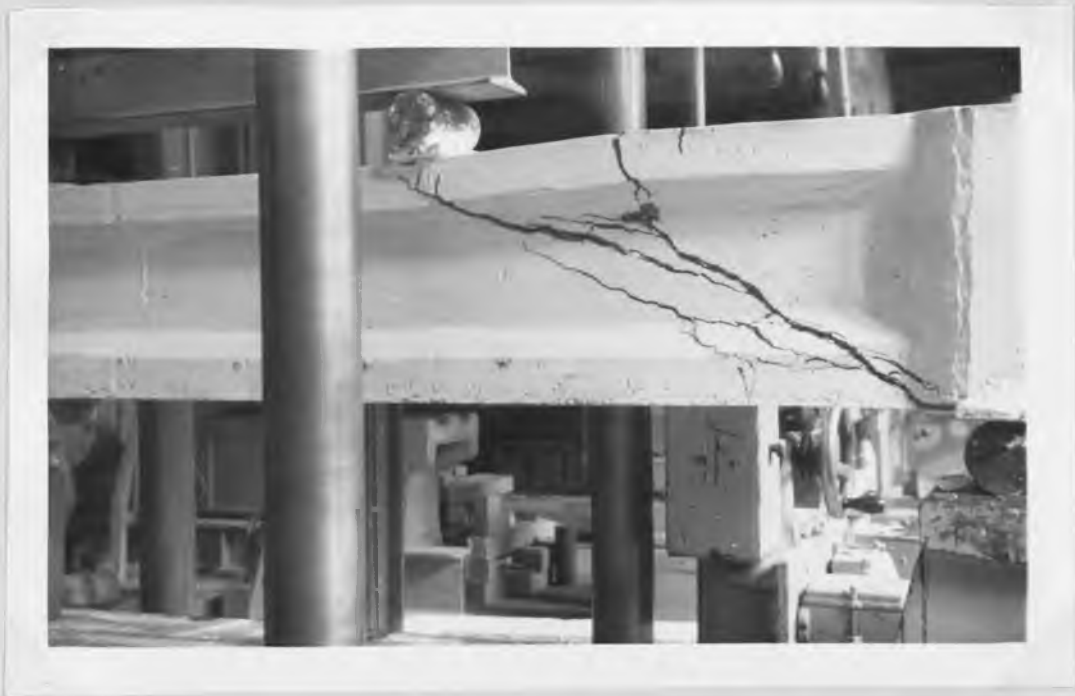
Plate 13 Failure by crushing of concrete within the web
