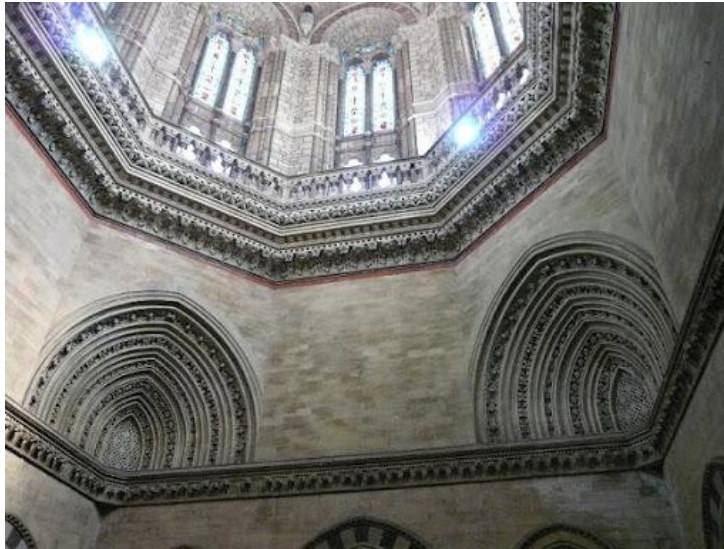
Fig. 33 CST, head of stairwell and base of drum with glass
