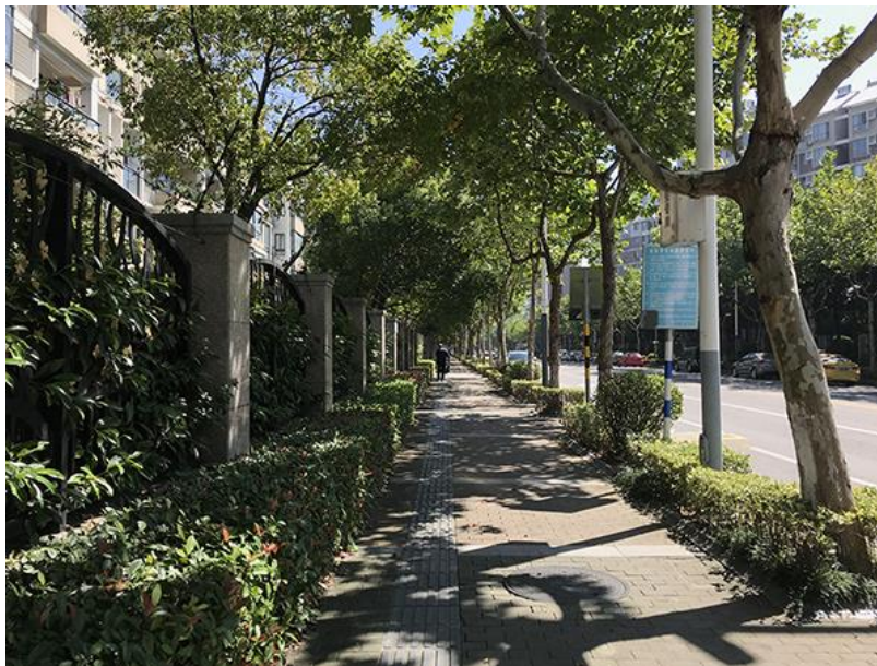
Figure 8.8 The pavement on Huashan Road (photo taken in 2017).
