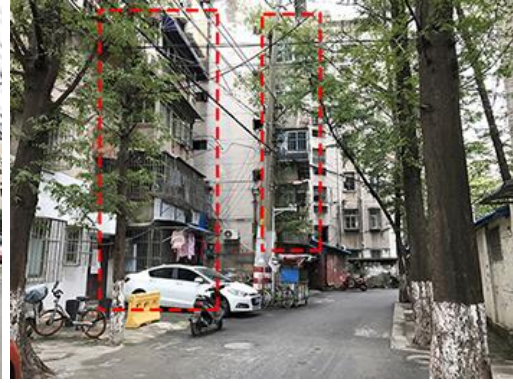
Figure 6.10f Balconies enclosed by residents.
