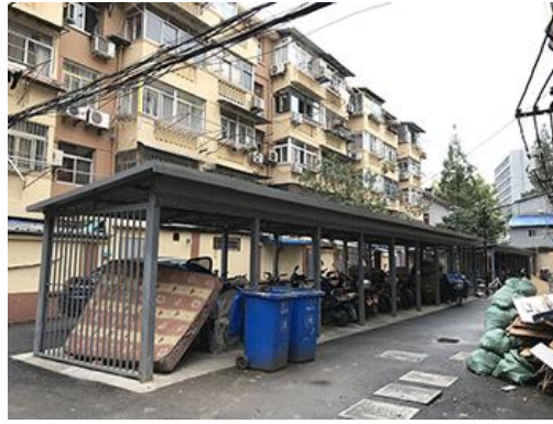
Figure 6.18d Building bicycle sheds.
