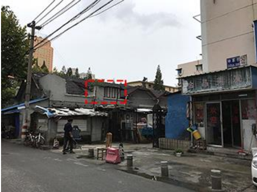
Figure 6.10a An extension on the roof.
