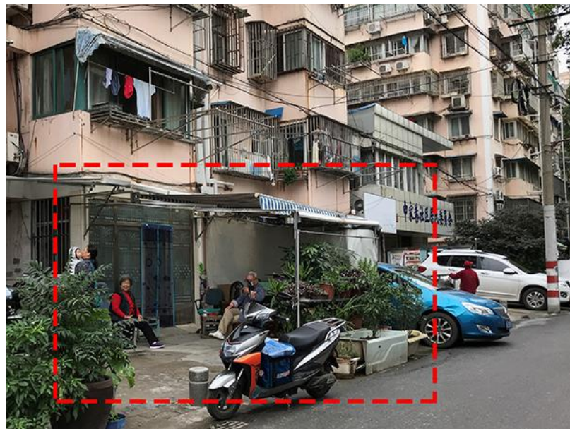
Figure 6.12 A extension was built by residents (photo taken in 2017).
