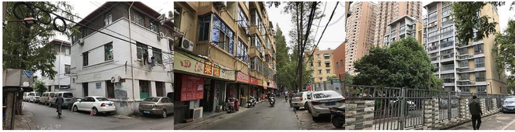
6.3a Historical buildings 6.3b Buildings built in the 1980s 6.3c High-rise buildings Figure 6.3 Three main building typologies in Shenjiaxiang community (photo taken in 2017).
