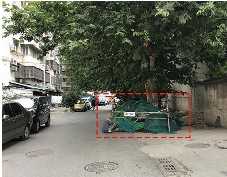
Figure 6.19 The stacking area for tools and materials is located at the edge of the street and does not affect peoples' movements and daily lives (photo taken in 2017).
