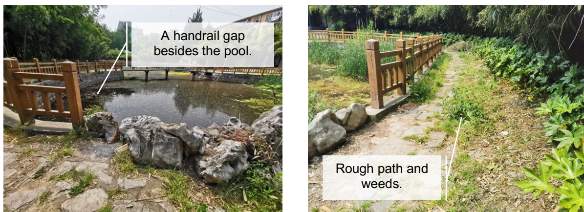
Figure 7.13 The abandoned yard in Case 1 community
