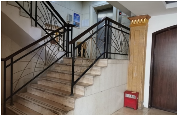
a. Steps in front of the lift
