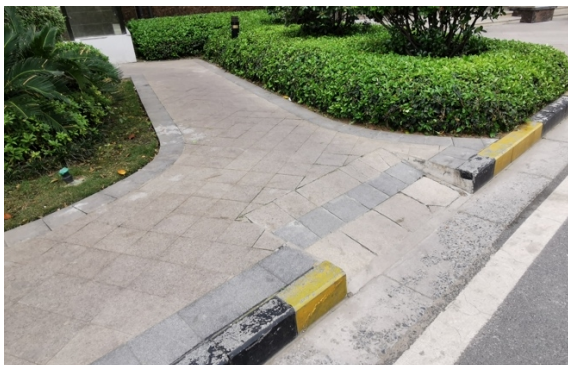
e. The height transition between the road and the pavement
