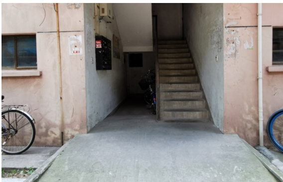
g. Ramp into the building entrance
