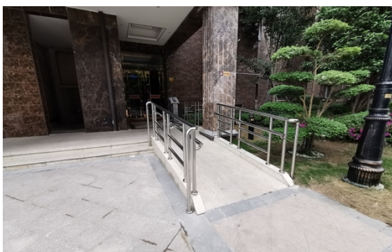
g. The ramp and handrails at the entrance of the building
