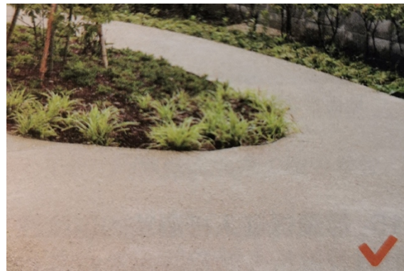
Smooth and uniform cement is suitable for pavement surfaces.
