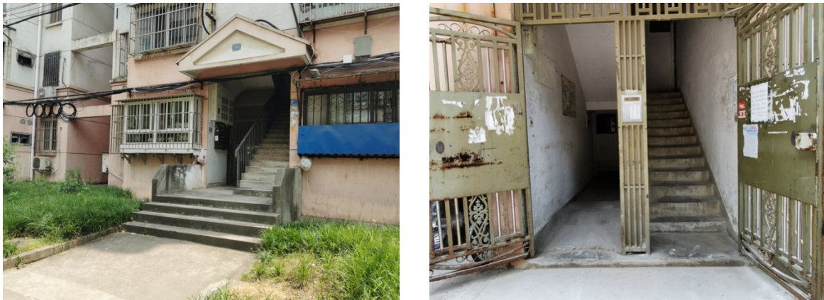
Figure 6.2 Building entrances in Case 1
