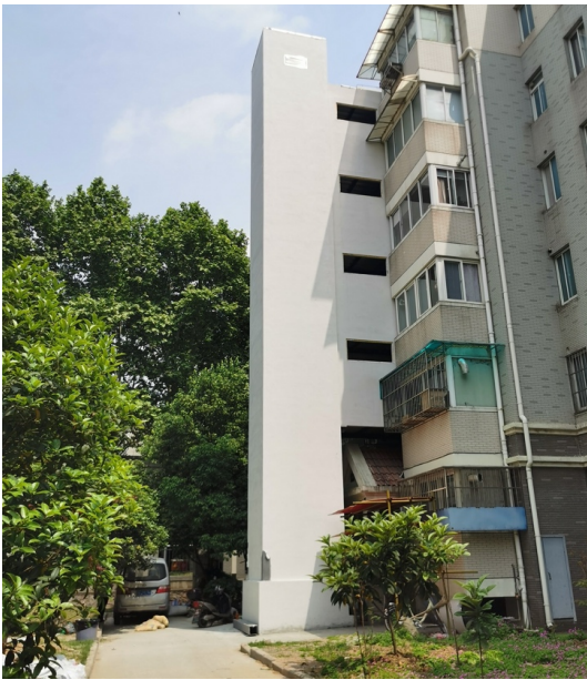
Figure 7.5 The new added lift in Case 1
