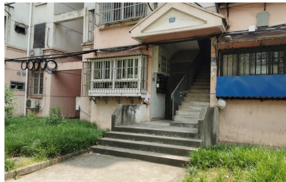
f. Steps into the building entrance
