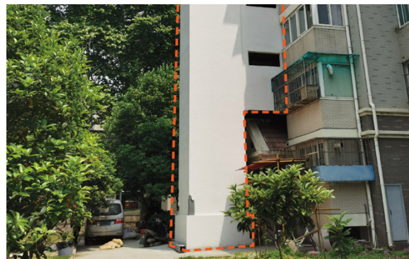
h. New lift which was added
