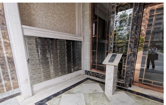
h. Access control system and post boxes in the residential building entrance
