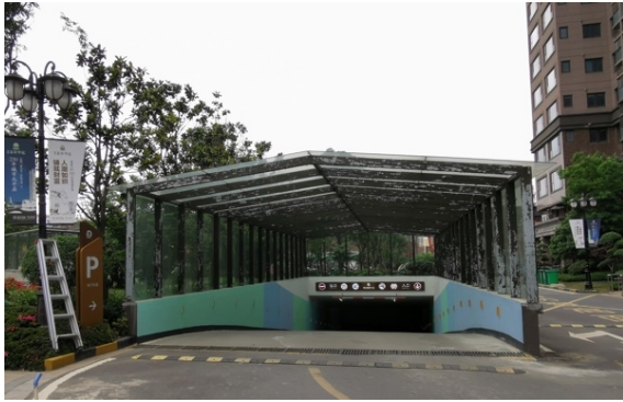
a. The entrance of underground parking
