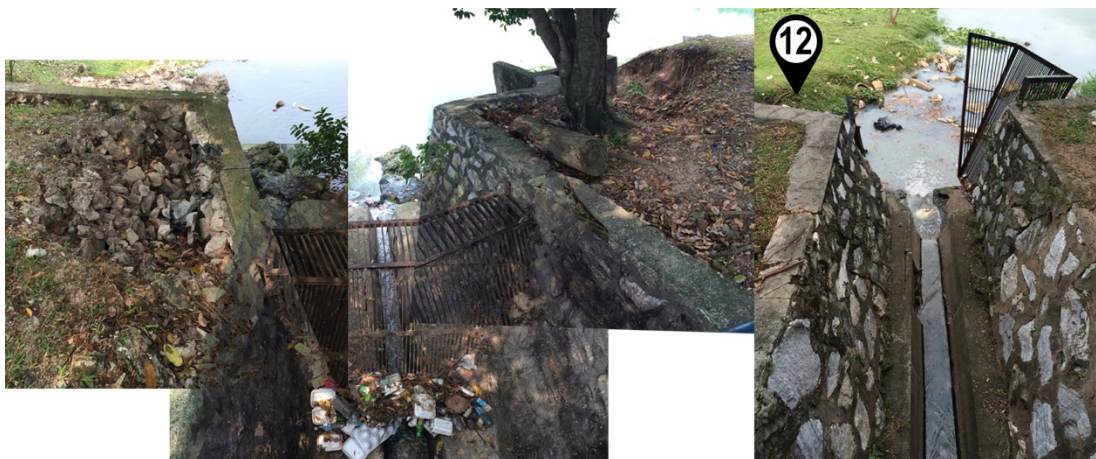
Figure 6.36 Photographic collages of two inlets that allow water to flow from the neighbourhood. The one on the right is node 12
