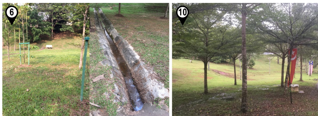
Figure 6.41 Photographs of node 6 (left) and node 10 (right) illustrate two maintenance issues, the untrimmed grass with polluted drain, and waterlogging
