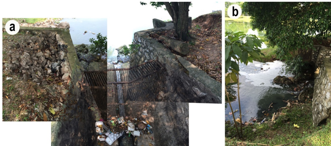
Figure 6.46 Photographic collages node 8 of the open drain that shows the deep ground holes (a) and untrimmed tree at the drain edges
