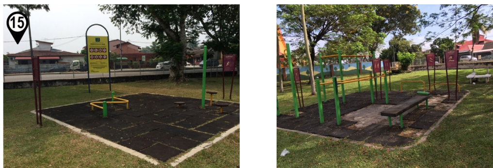
Figure 6.31 Photographic image of outdoor gym station, node 15, that shows the poor condition of the equipment and some damage to the interlocking rubber mats
