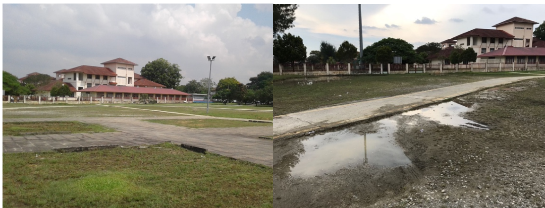
Figure 6.38 Original of node 2 portrays the issues of waterlogging that exist at so many spots within this open space
