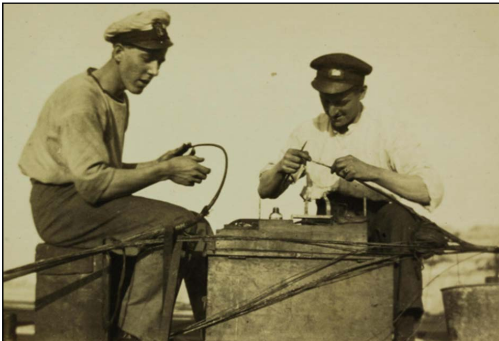
Fig 6.6 The Cable Jointer and his assistant preparing to splice two lengths of submarine cable at a jointer's bench. This photograph was taken in 1910 but the technique used was identical to that in 1883. Only the hats would have been different! PK Archives photo 0400
