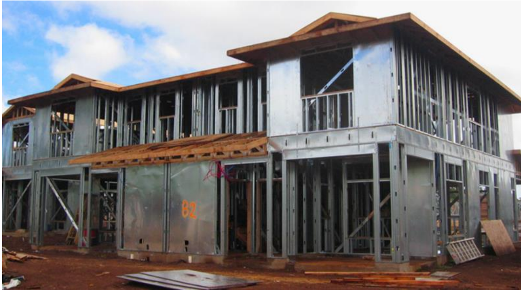
Figure 1.2 Typical CFS framed building with steel sheathed shear walls (photo courtesy of J.Ellis, Simpson-Tie Co. Inc.)
