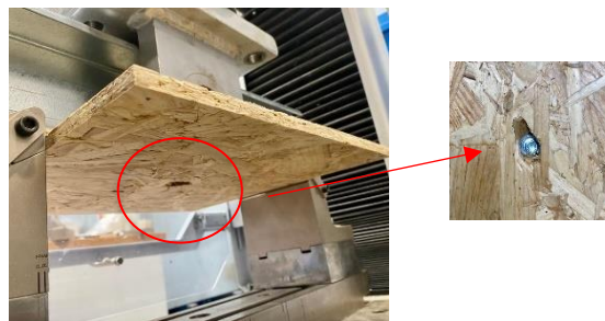
Figure 4.17 Typical failure mode captured from the pull-out tests
