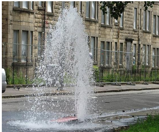
Figure 1-1 Image of underground potable water leakage (Water matters UK.2013)
