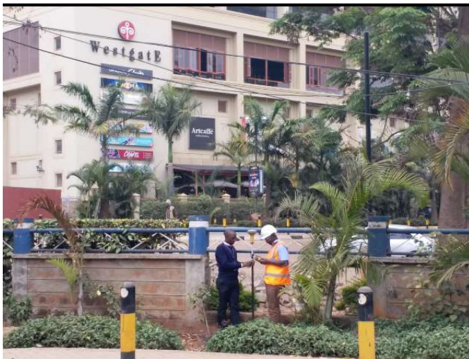
Figure 71. Survey in progress at the Westgate Shopping Mall flooding hotspot showing a breach of the shopping mall fence line during the March 2018 flooding event to allow the passage of floodwater – brick rubble can be seen visible behind the gaping hole in fence wall in the background.
