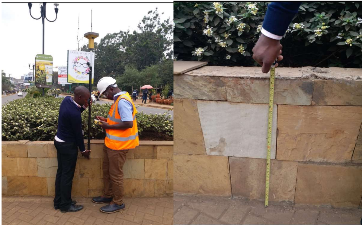
Figure 72. Measurement of flood historic flood depth levels at flooding hotspot site.
