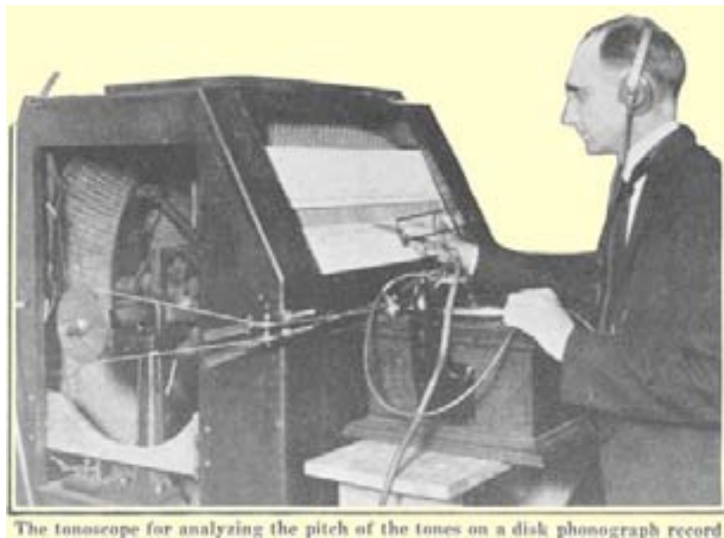
Figure 2.3. A figure showing Seashore working on the tonoscope for creating music stimuli. Image from Cary (1992).
