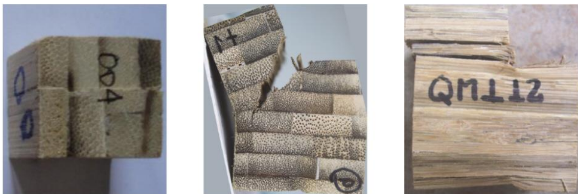
Figure 2. 19: left – perpendicular shear failure reported by Kariuki (2018) , centre and right – perpendicular shear failures reported by Estrada, Linero and Takeuchi (2019) .
