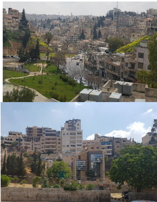
Figure 54: Left: 7 Hills Skate Park from the Jabal Amman Side, Showing Prince Mohammed St. Leading to Downtown (Taken from Al-Imam Ahmed Bin Hanbal Street); Right: View from Prince Mohemmed St. Showing Jabal Lwebde Houses that Overlook the Park. Source: Author, 2019.
