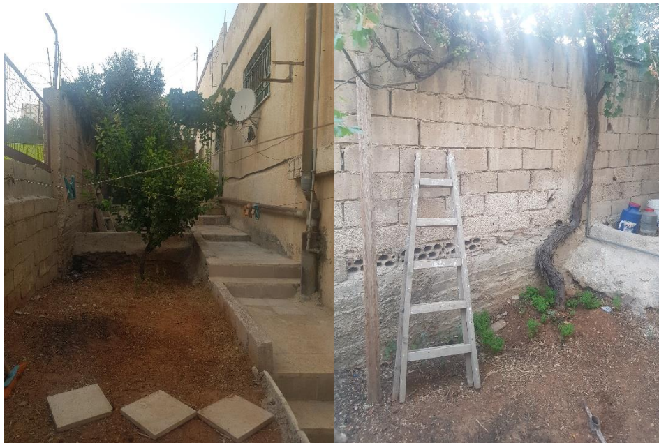
Figure 110: Akram's Designated Path, the Ladder, and the Vine at the Third Platform
