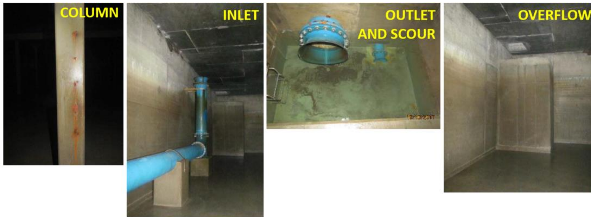
Figure 5.12 – A schematic of B6 SR and a few photos displaying some of the internal details of the SR.
