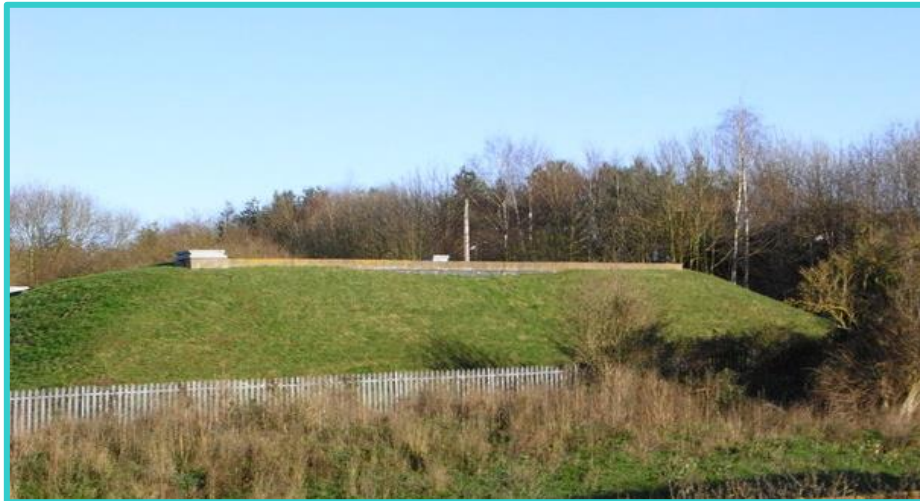
Figure 2.3 – An underground service reservoir with a grass covered roof.
