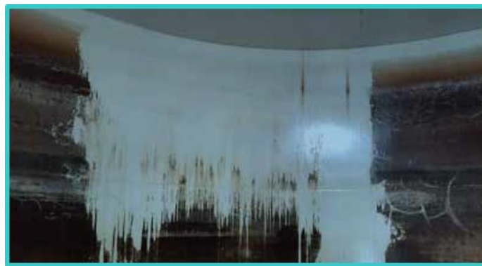
Figure 2.13 – An example of the biocide solution used to clean service reservoirs in practice. Source: USEPA.
