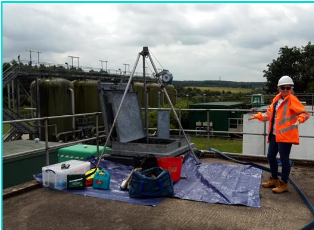
Figure a – An example of what a hygienic SR set up should look like.
