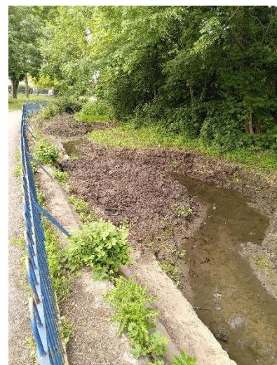
Image 23 - During early stages of the restoration project - Deflectors in place
