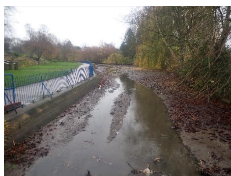
Image 20 - Photo of Osbaldwick beck from bridge after partial removal of the weirs
