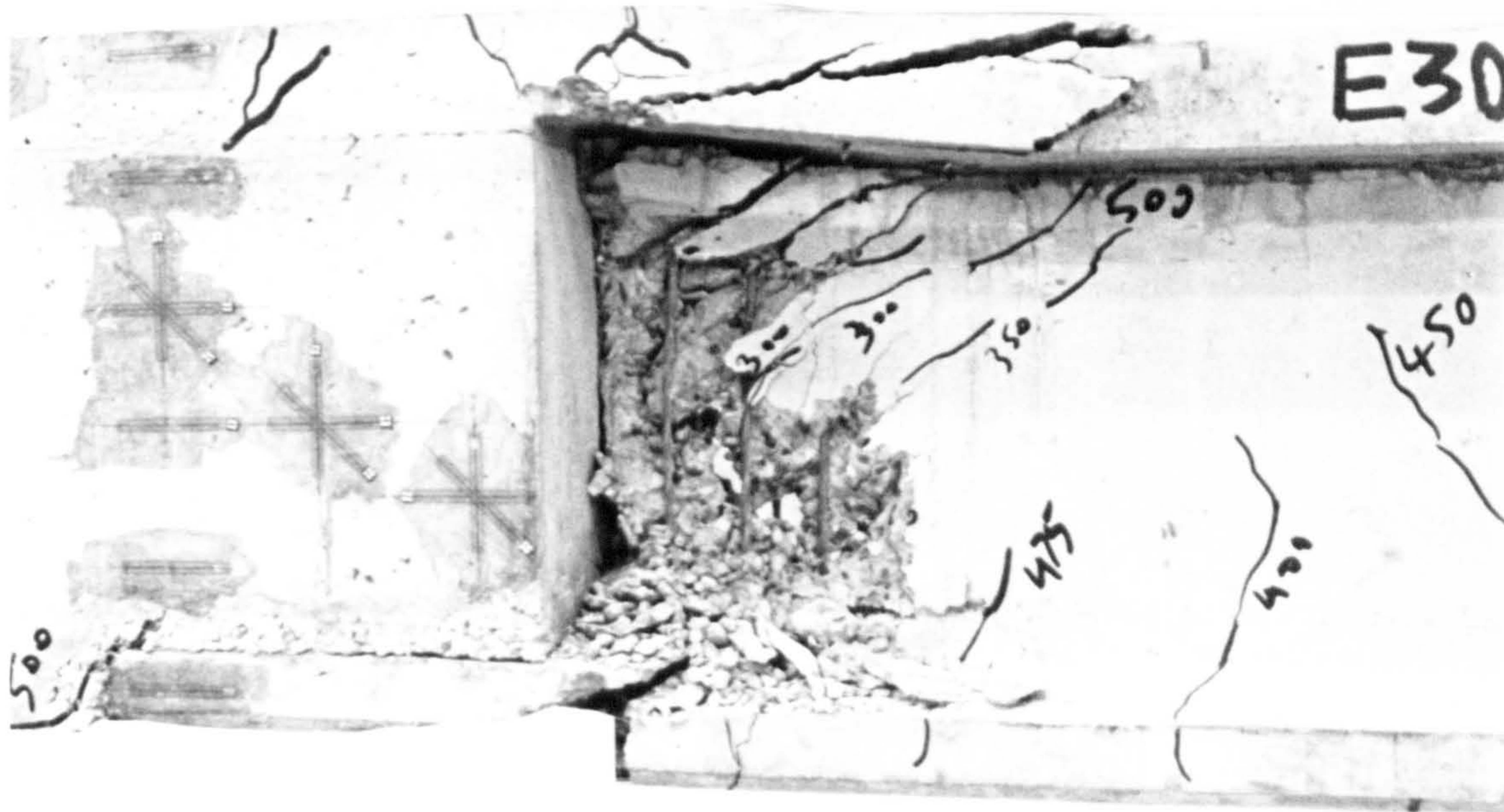
Plate 5.7 Elimination of Dowel action by Sleeving the Bars ( With Nib Stirrups) Condition in The Connection After Failure
