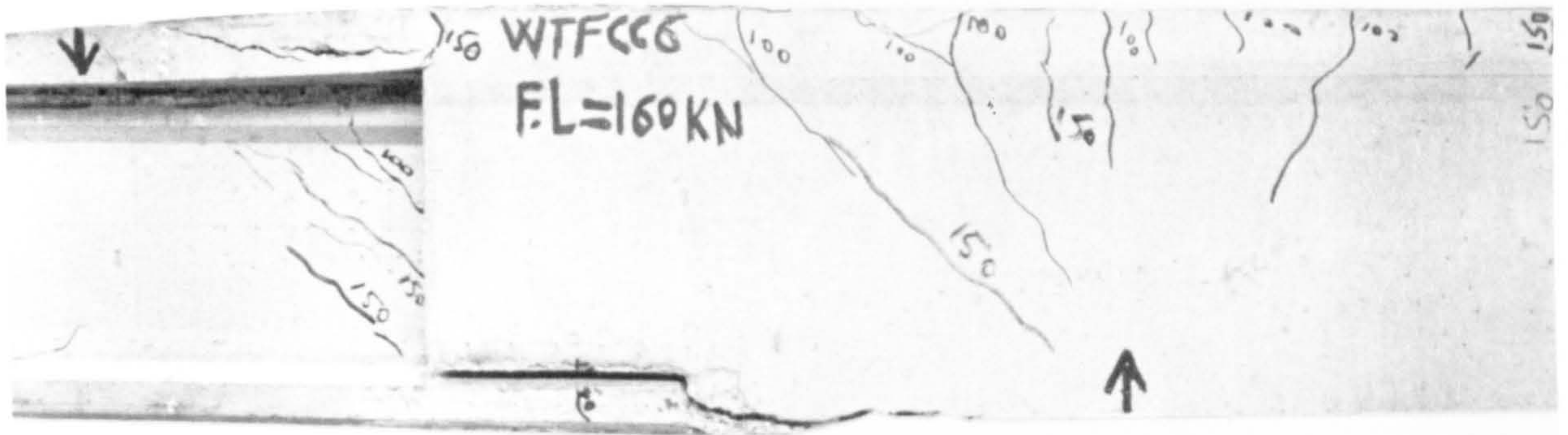
Plate 6.5 Elimination of Top Flanges (The Connection Failure)
