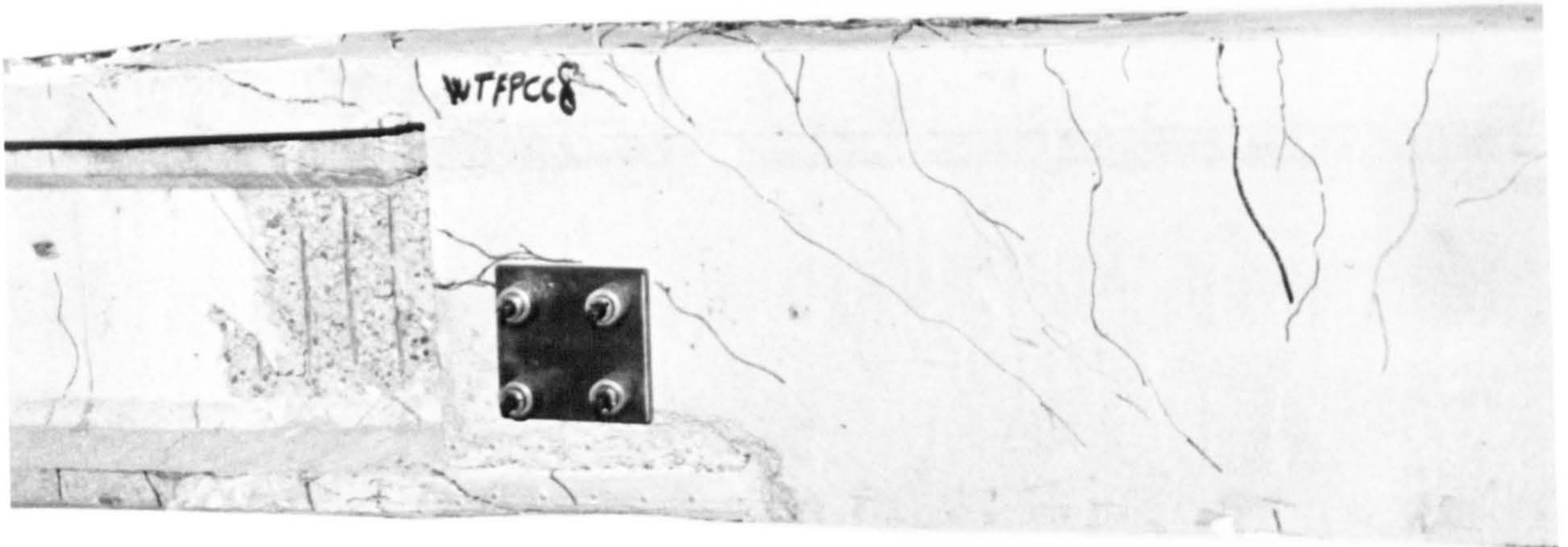
Plate 6.6 Provision of Transverse Prestressing (No Top Flange) Condition in The Connection After Failure
