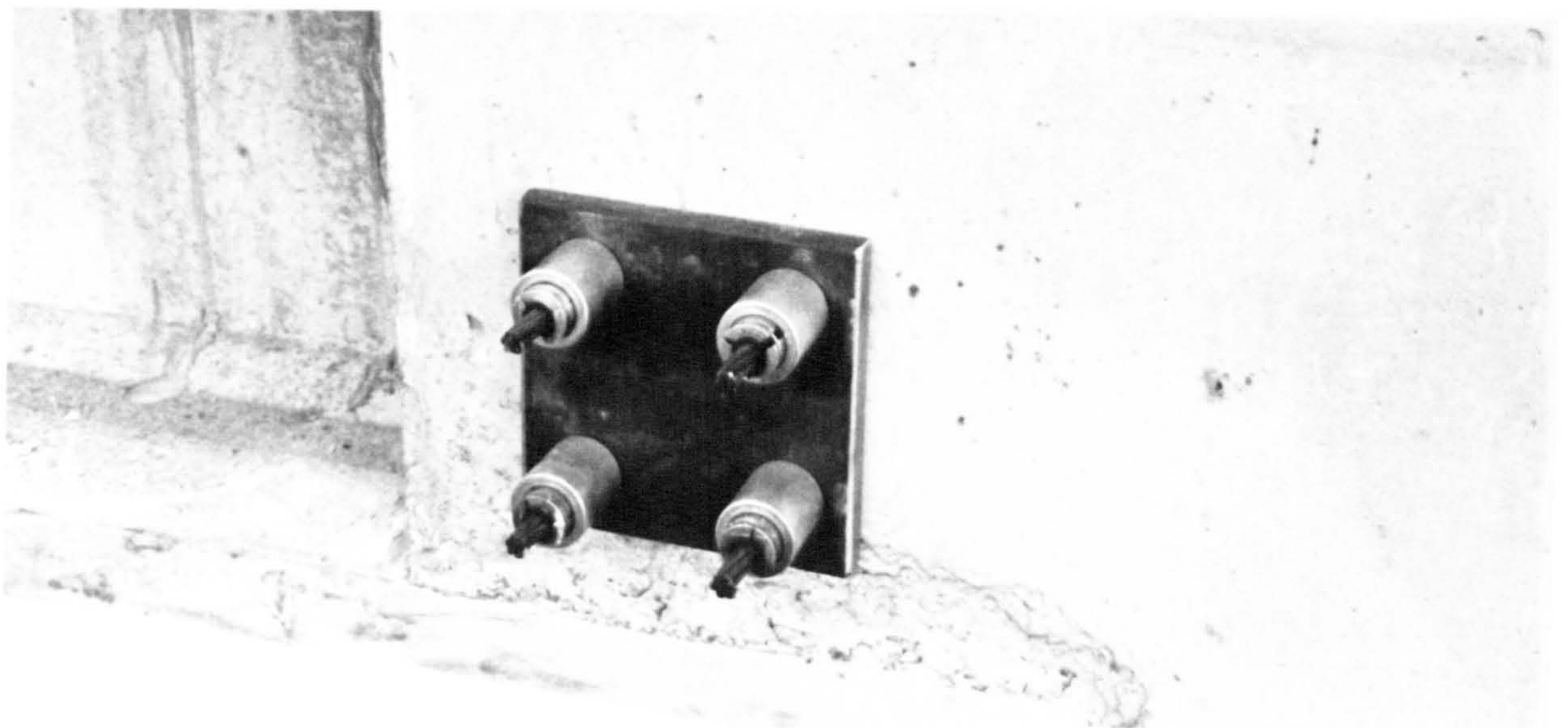
Plate 3.3 Transverse Prestressing at the Connection
