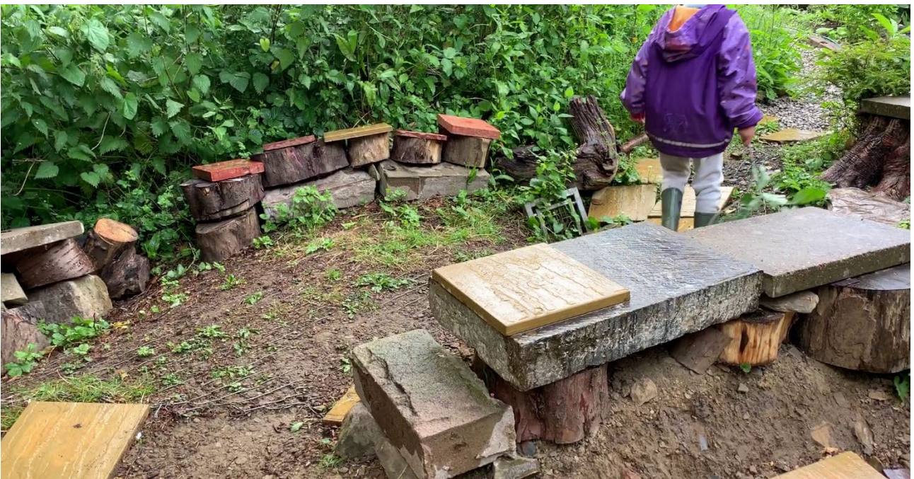
Figure 6.38. A seating area made from materials found around the site, including cut logs, paving slabs and stone.
