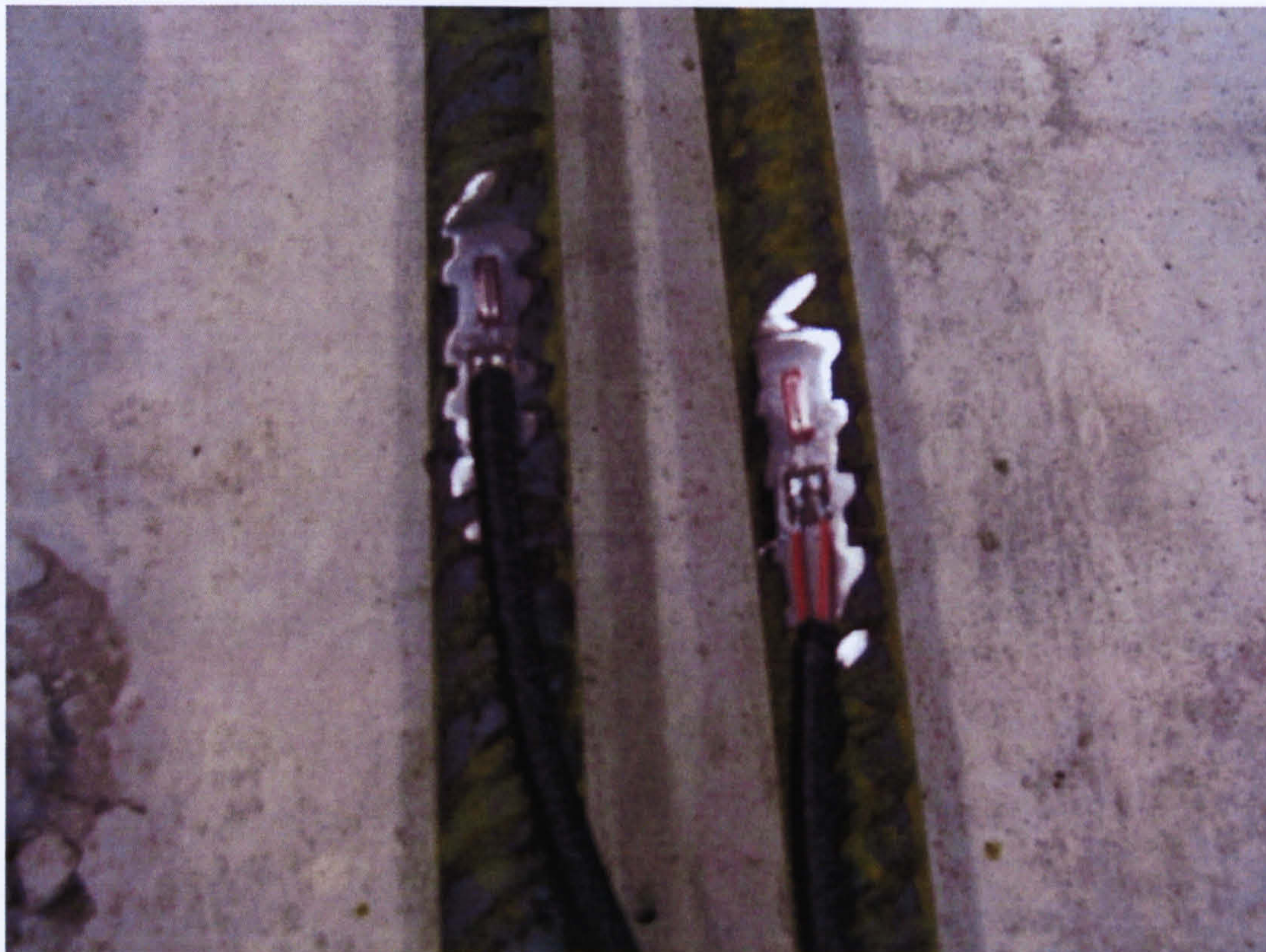
(a) Strain gauges placed at centre of transverse reinforcement
