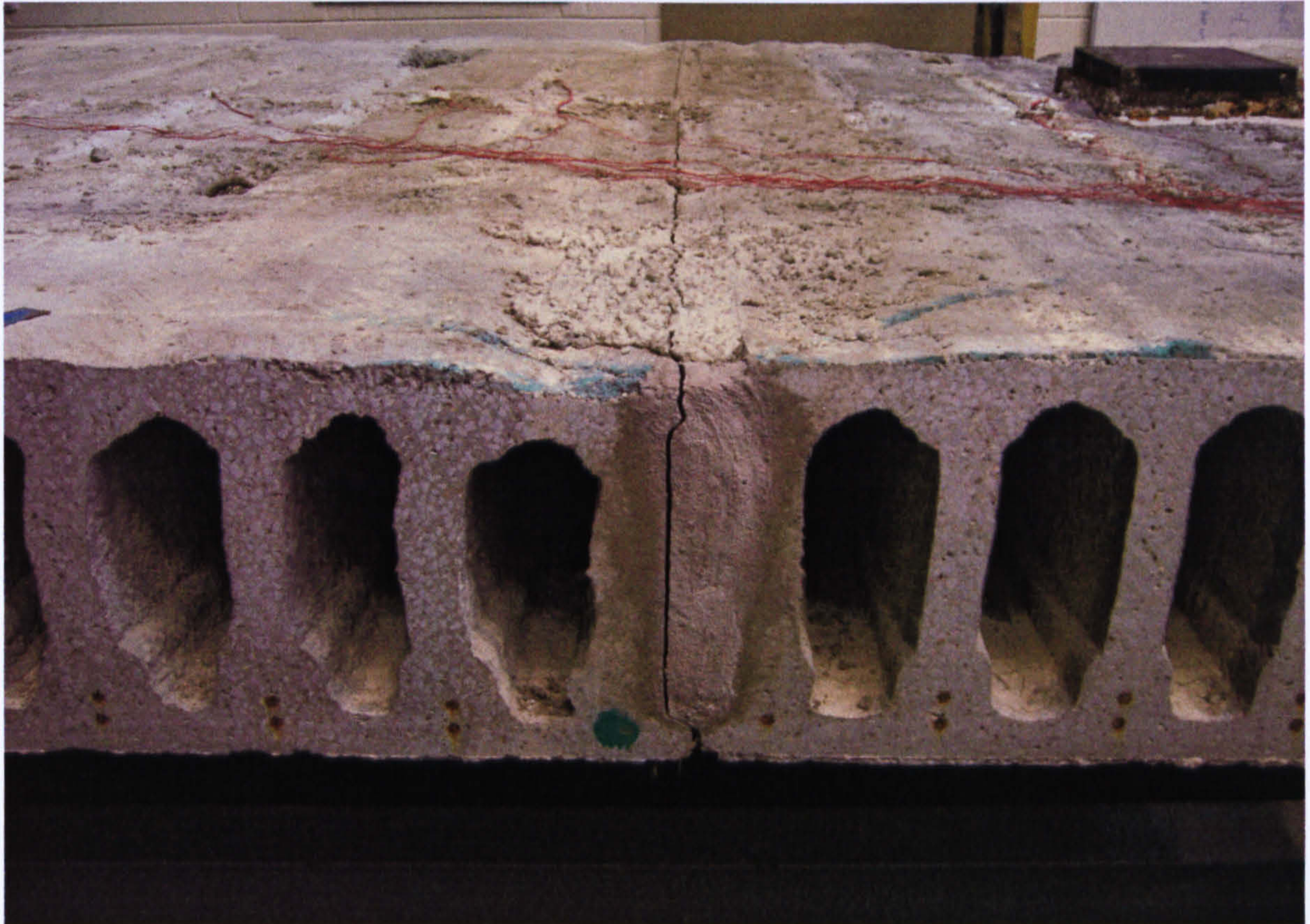
Figure 4.40: Tensile cracks in In-situ concrete of CB-5
