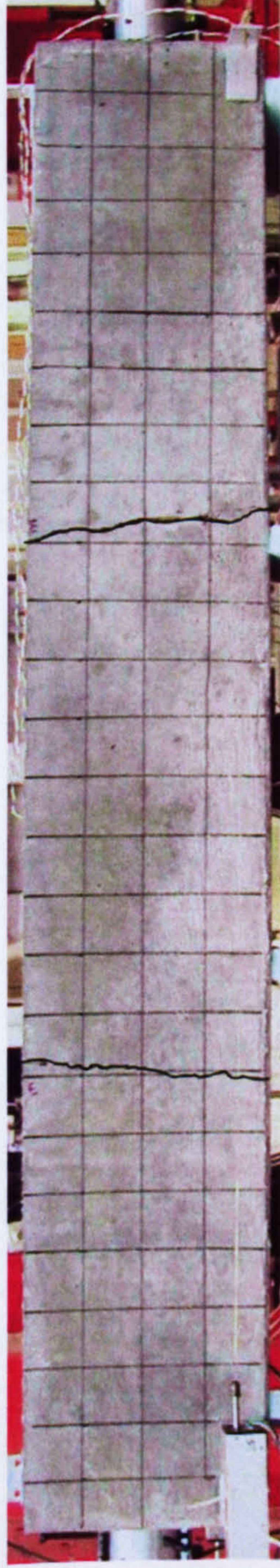
(a) Crack pattern of tested specimen
