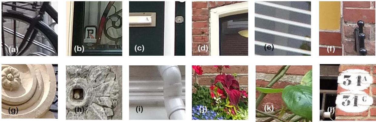
Figure 4-4: Images depicting various 'non-crack' objects included in the masonry dataset for the training of the classification network.
