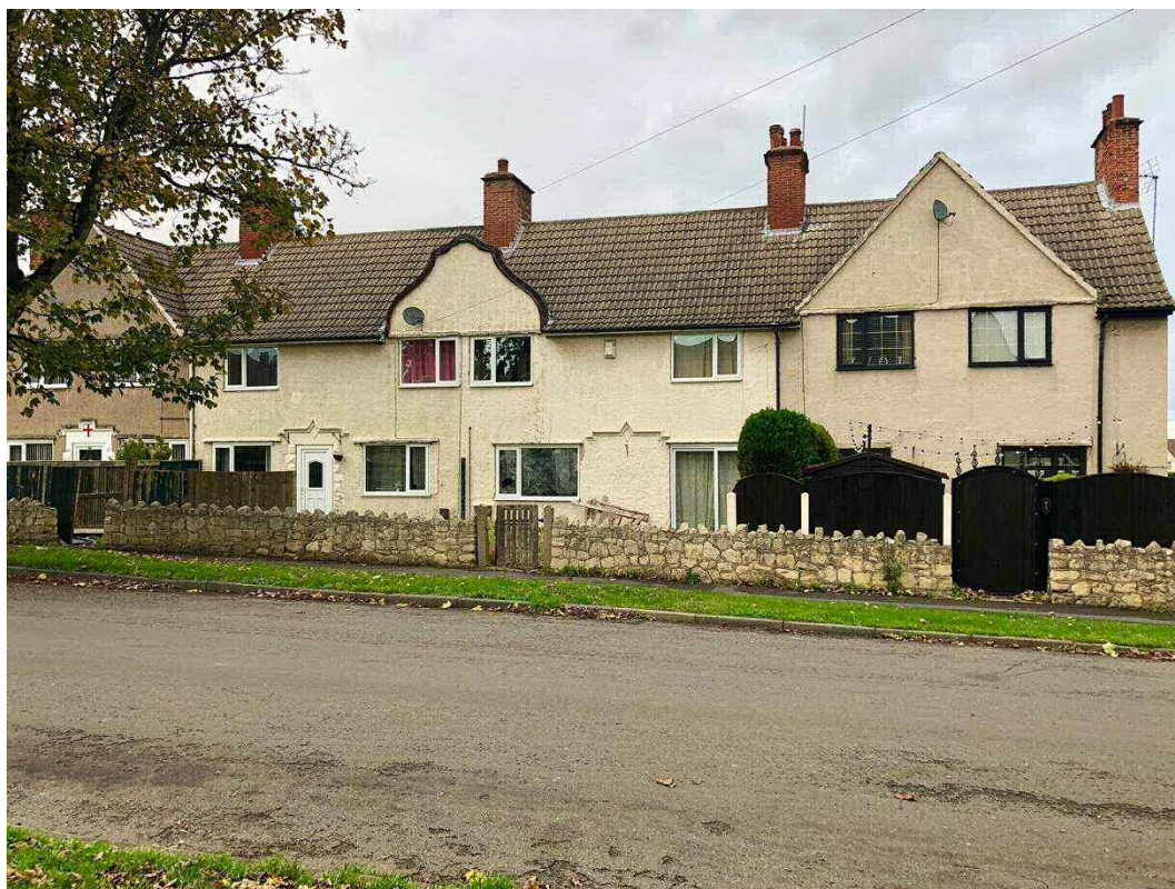
Fig. 45: Houses on West Avenue, featuring a blocked-up front door and implying a main access route from the open square to the rear. A patio door may have provided additional access and permitted more light into the main living spaces. © Author.
