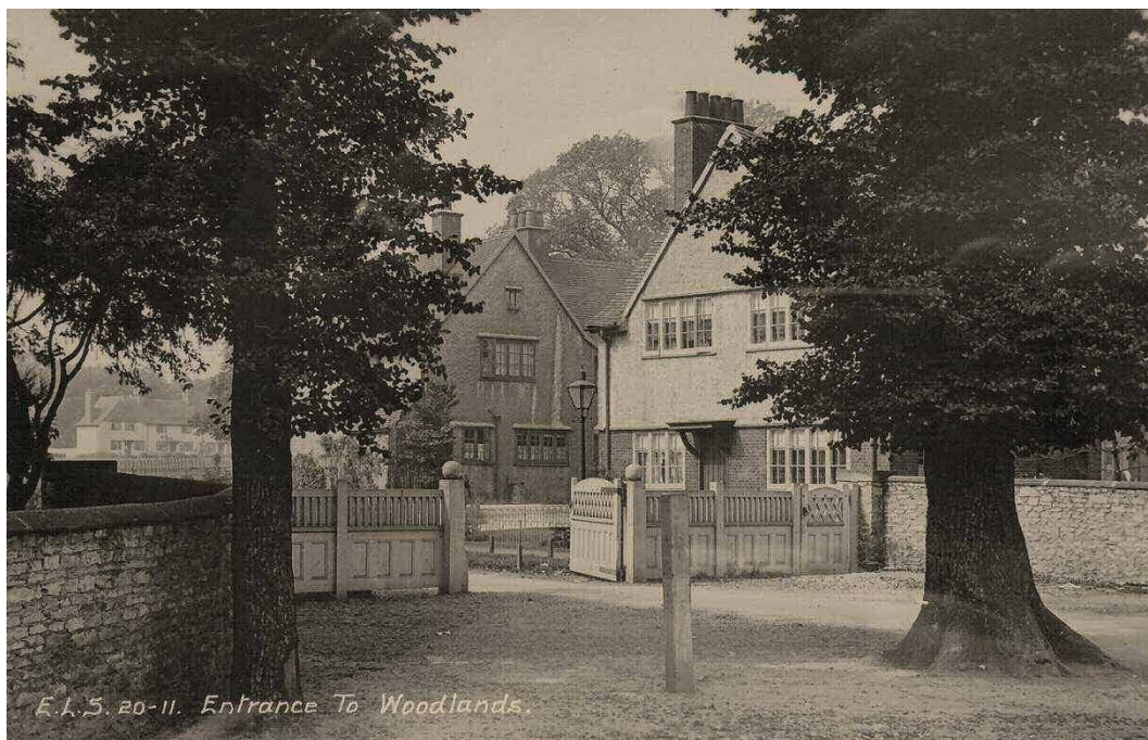
Fig. 40: Early-twentieth-century photograph by E. L. Scrivens, showing the former gated entrance into the Park from Great North Road, with one of a pair of 'lodge' houses to the right. Courtesy of WCHA.
