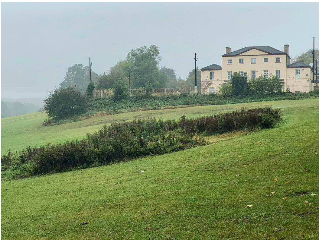
Fig. 34: Woodlands Mansion (as it was originally known, later becoming the Brodsworth Club or Institute, surviving now as Woodlands Park Club) with surrounding parkland south-east of the main village, both retained in the scheme. © Author.
