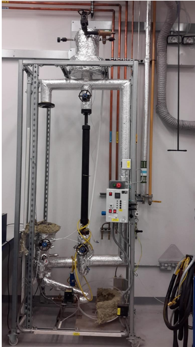
Figure 4-3: State of EES Experimental Rig
