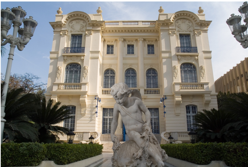
Figure 4 Mohamed Mahmoud Khalil Villa, No.1 Kafour Street. Barry Iverson
