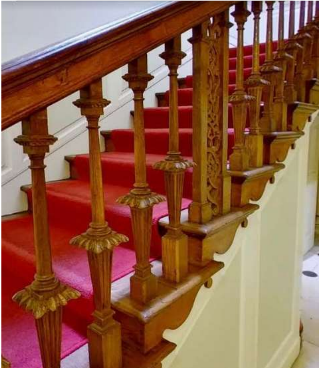
Figure 2.4: The best staircase at Cannon Hall showing square acanthus balusters, 1 st June 2021, photograph by author.
