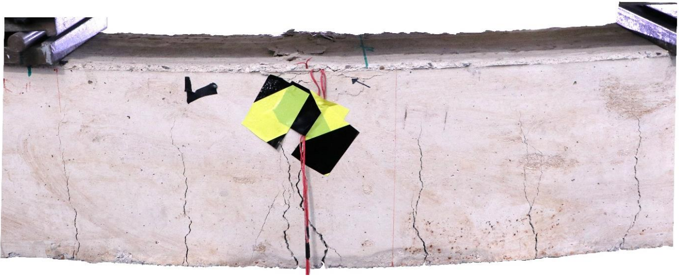
Figure 5.11 The mode of failure for control beam B-REF (crushing of concrete after the yielding of internal reinforcement).
