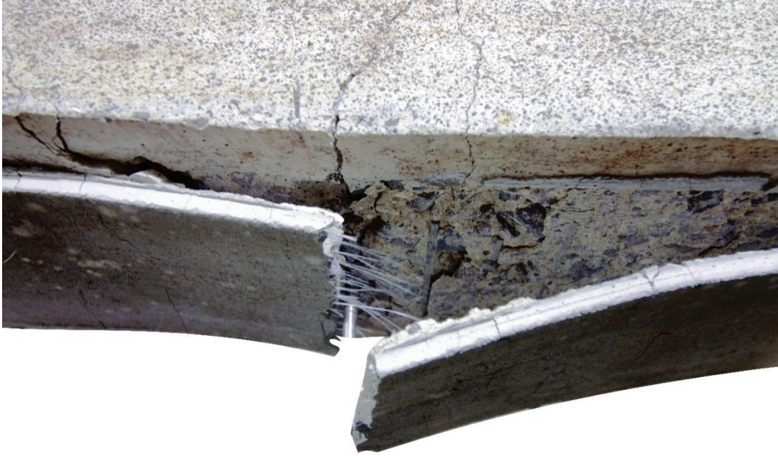
Figure 5.13 The mode of failure for beam B-S4-1 (rupture of steel textile).
