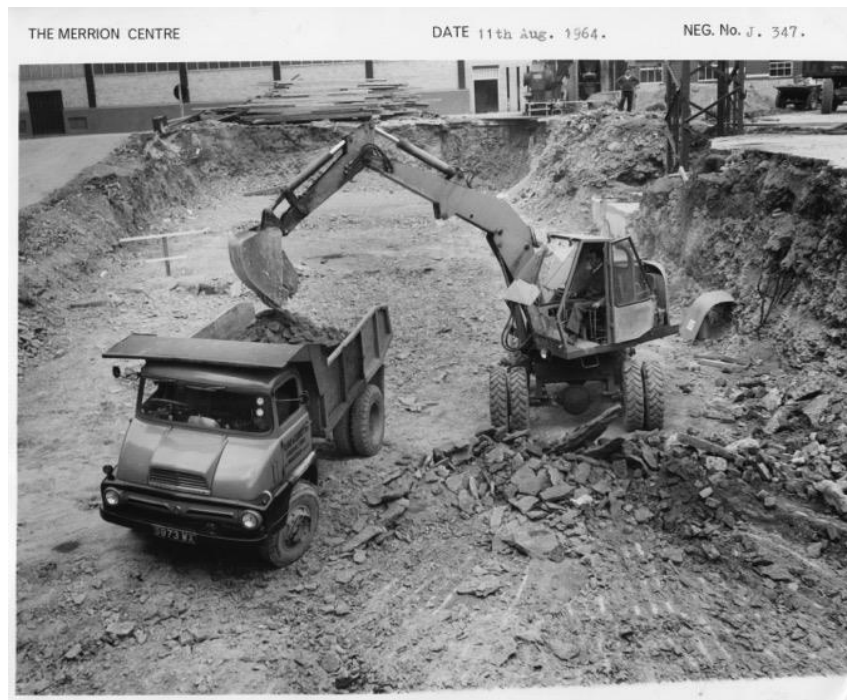
Fig 161. Construction of Merrion Centre,1964. [Photograph]. At: Town Centre Securities Archive
