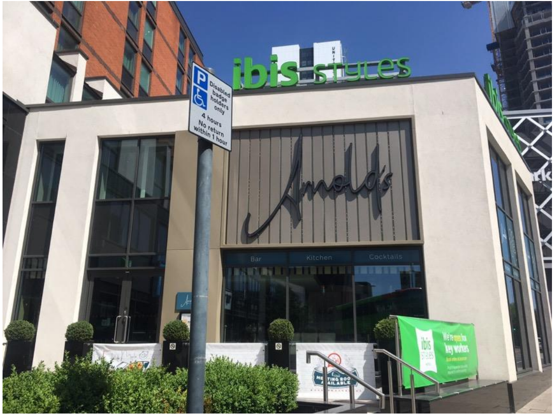
Fig 50. Stone, A. 2020. Arnold's , Merrion Centre. [Photography].
