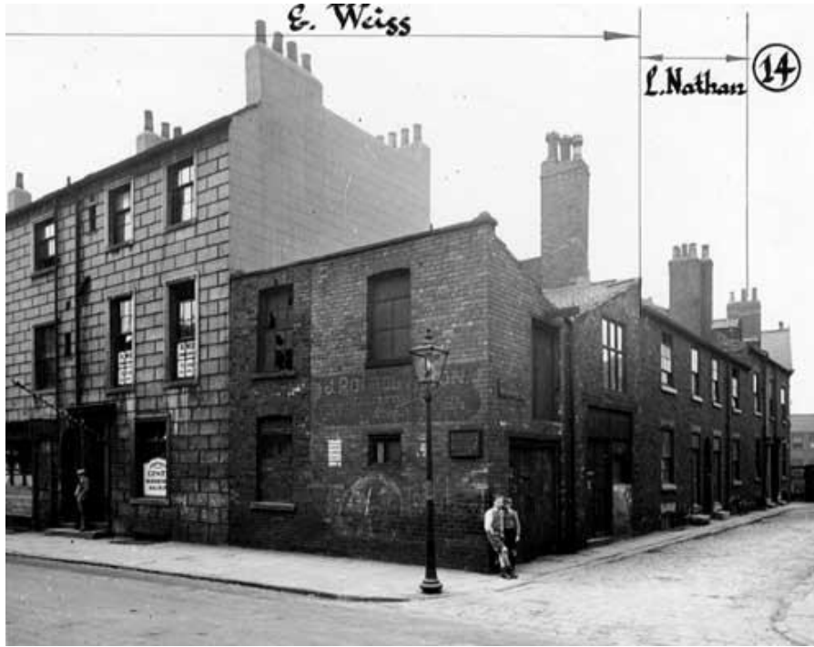
Fig 156. West Yorkshire Archive Services, Rockingham Street, 1946, Leodis https://www.leodis.net/viewimage/62309
