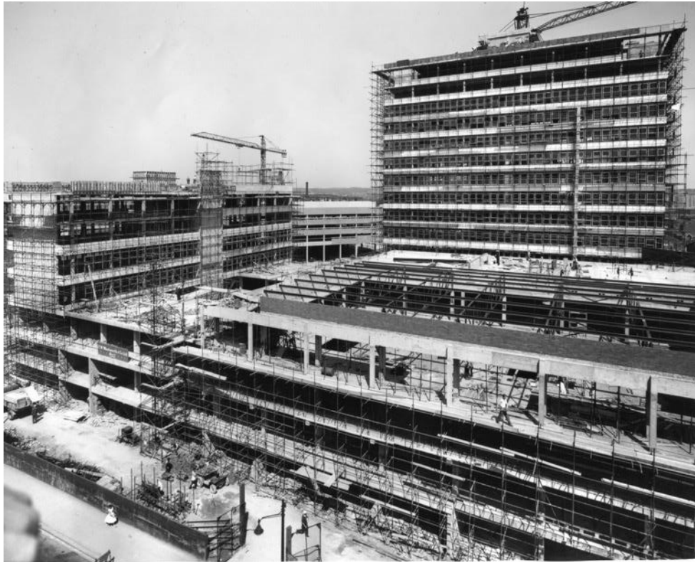
Fig 39. Merrion Centre Construction. 1962.[Photograph]. At: Leeds: Town Centre Securities Archive
