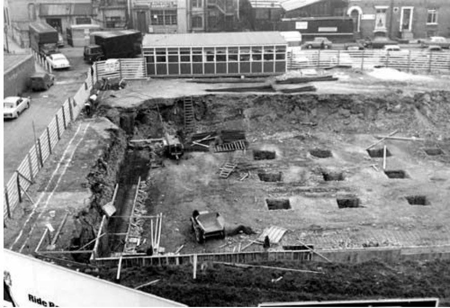
Fig 160. Brunswick Terrace/ Wade Passage excavation, 1965. [Photograph]. Leodis. https://www.leodis.net/
