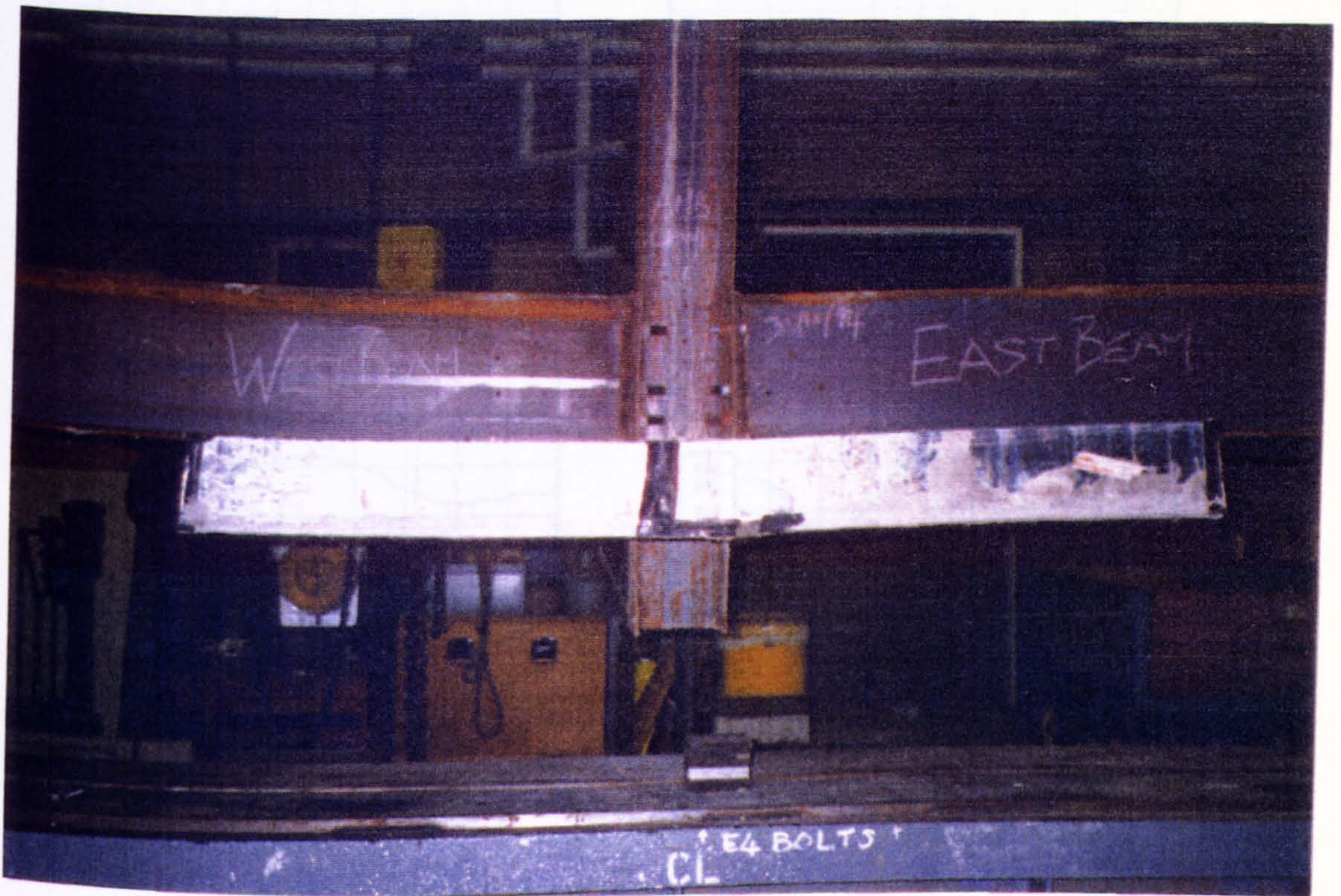
Figure 3.28. Ambient-Temperature Composite Connection Failure Mechanism
