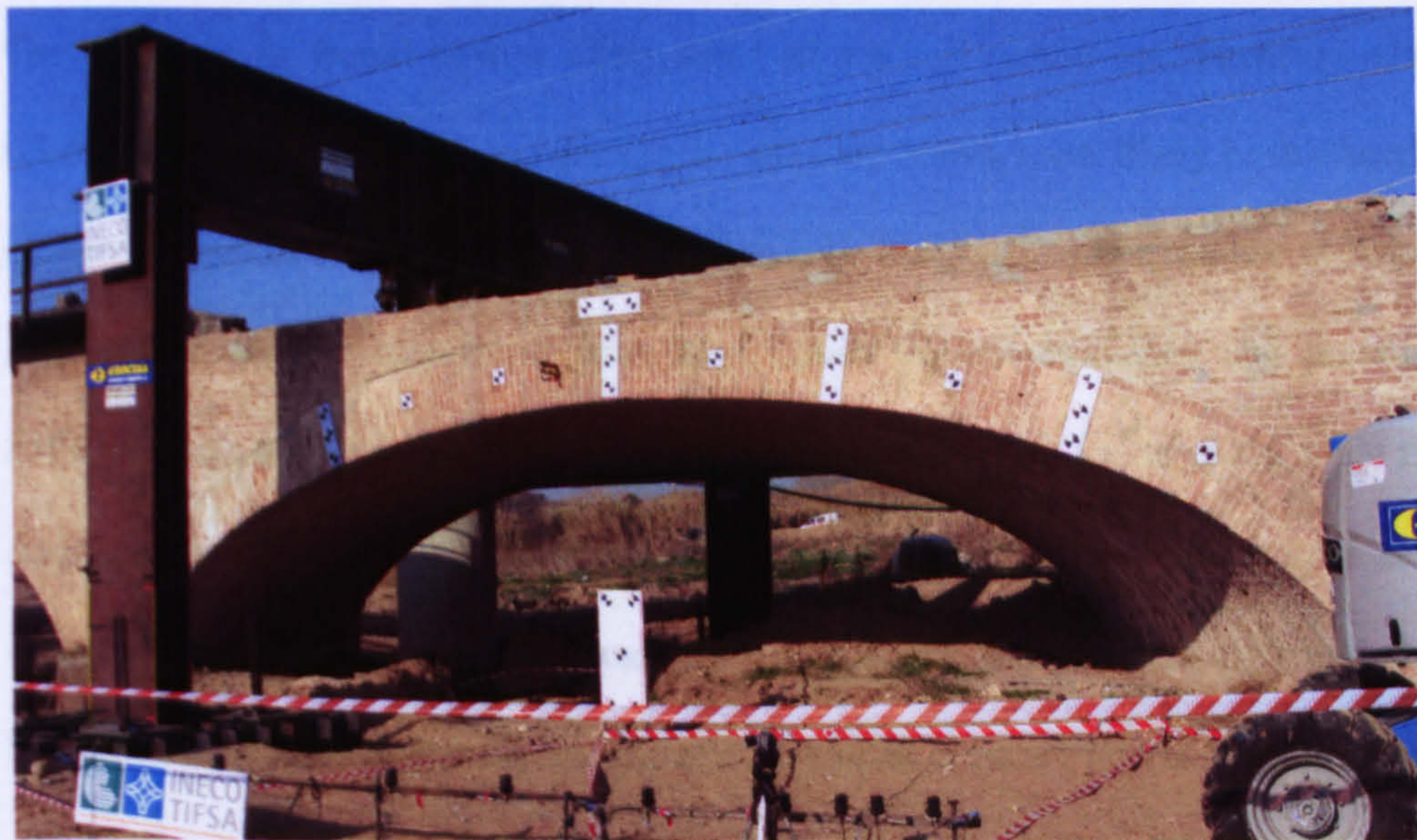
Figure 3-11 Field bridge test Barcelona 2005
