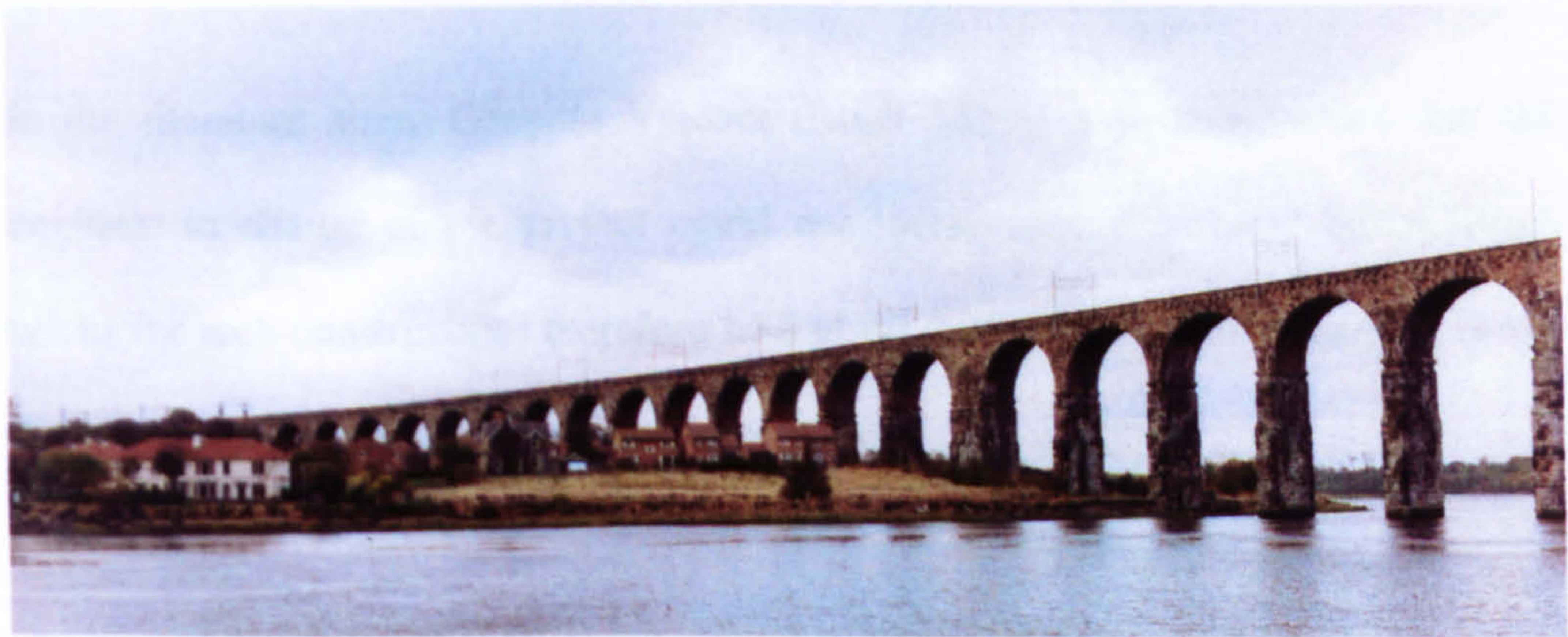
Figure 2-8 Royal Border Bridge (Courtesy of Network Rail)
