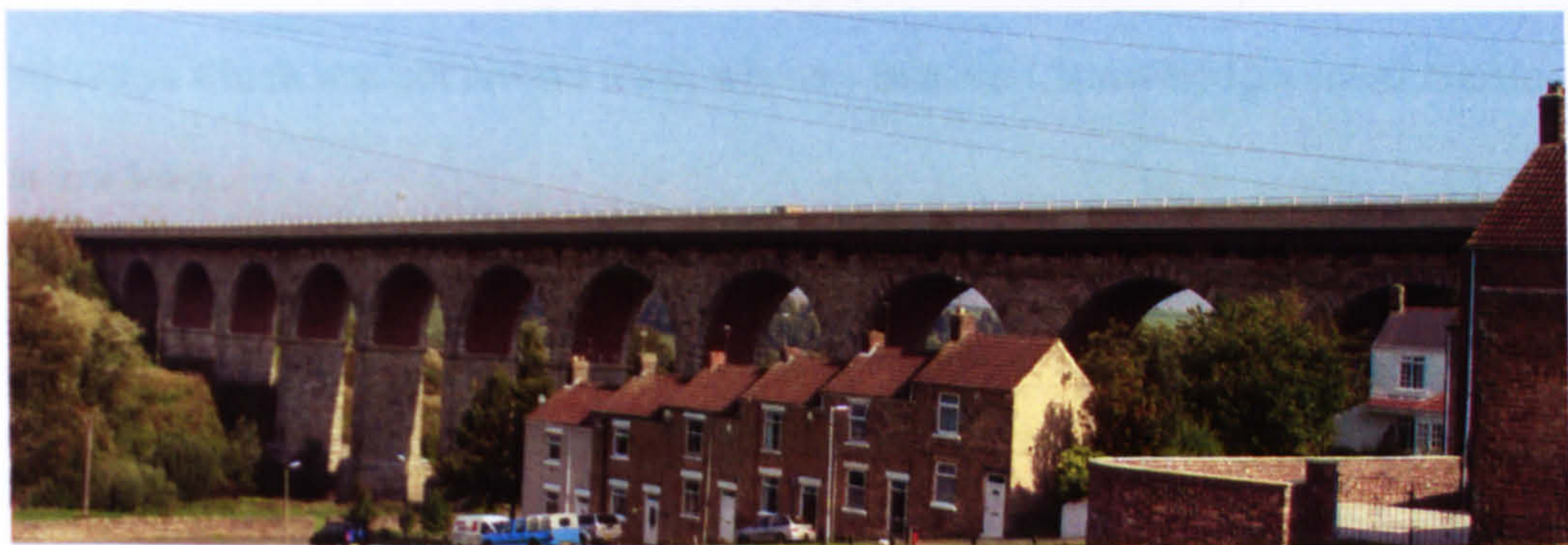
Figure 2-9 The 1848 bridge at Newton Cap, Bishop Auckland, Co. Durham
