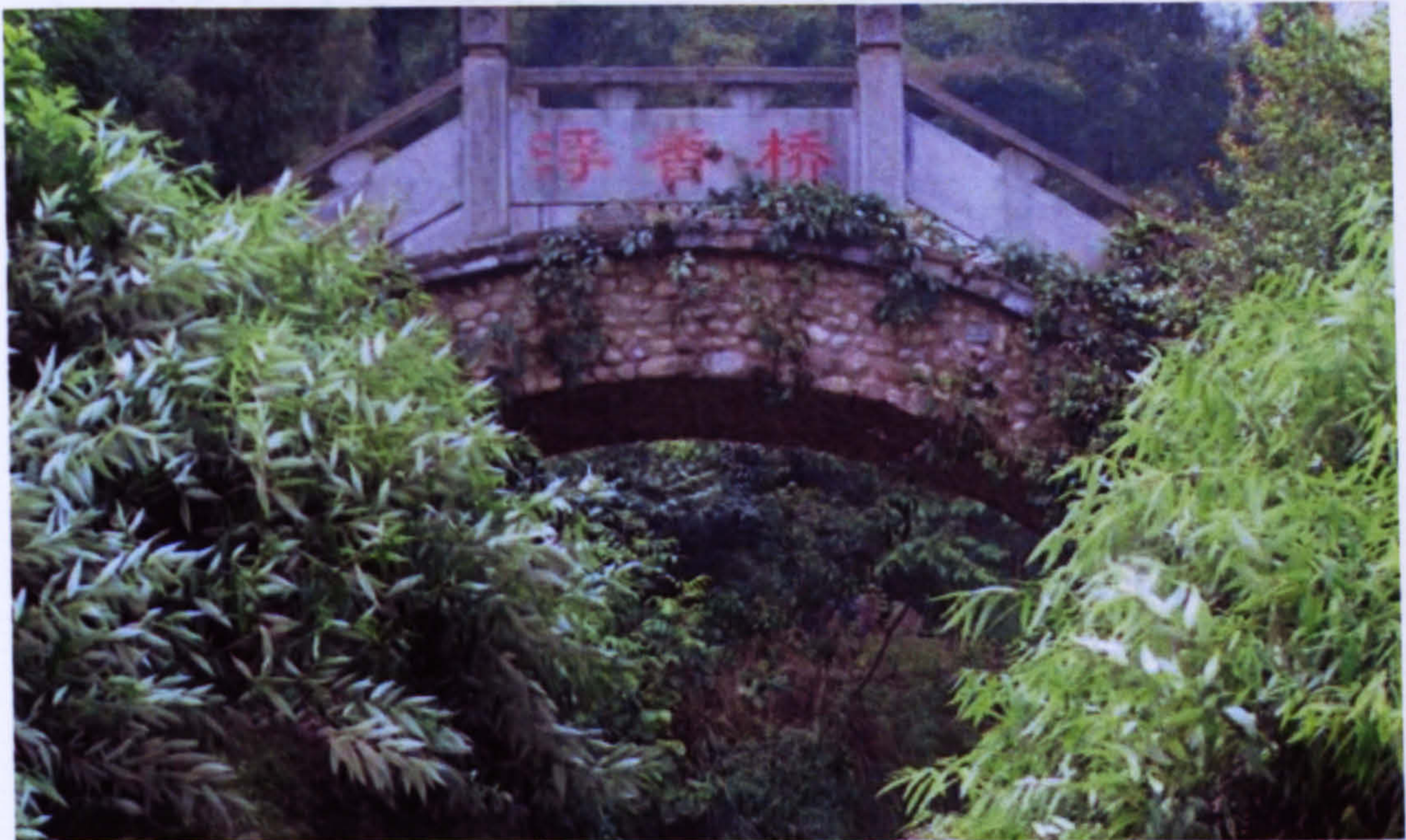
Figure 2-3 An arch bridge, Che Spring Reservation, Ye Chang, China
