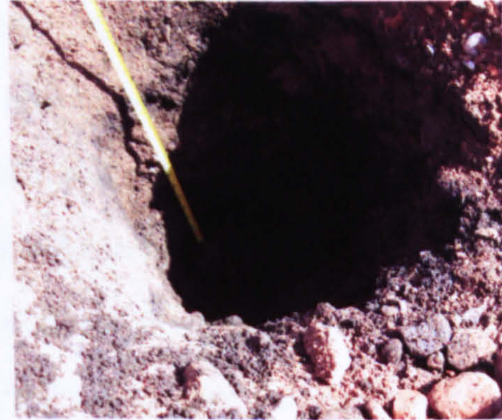
Figure 2-12 Trial pit in bridge TCC/20 (Courtesy of Network Rail)
