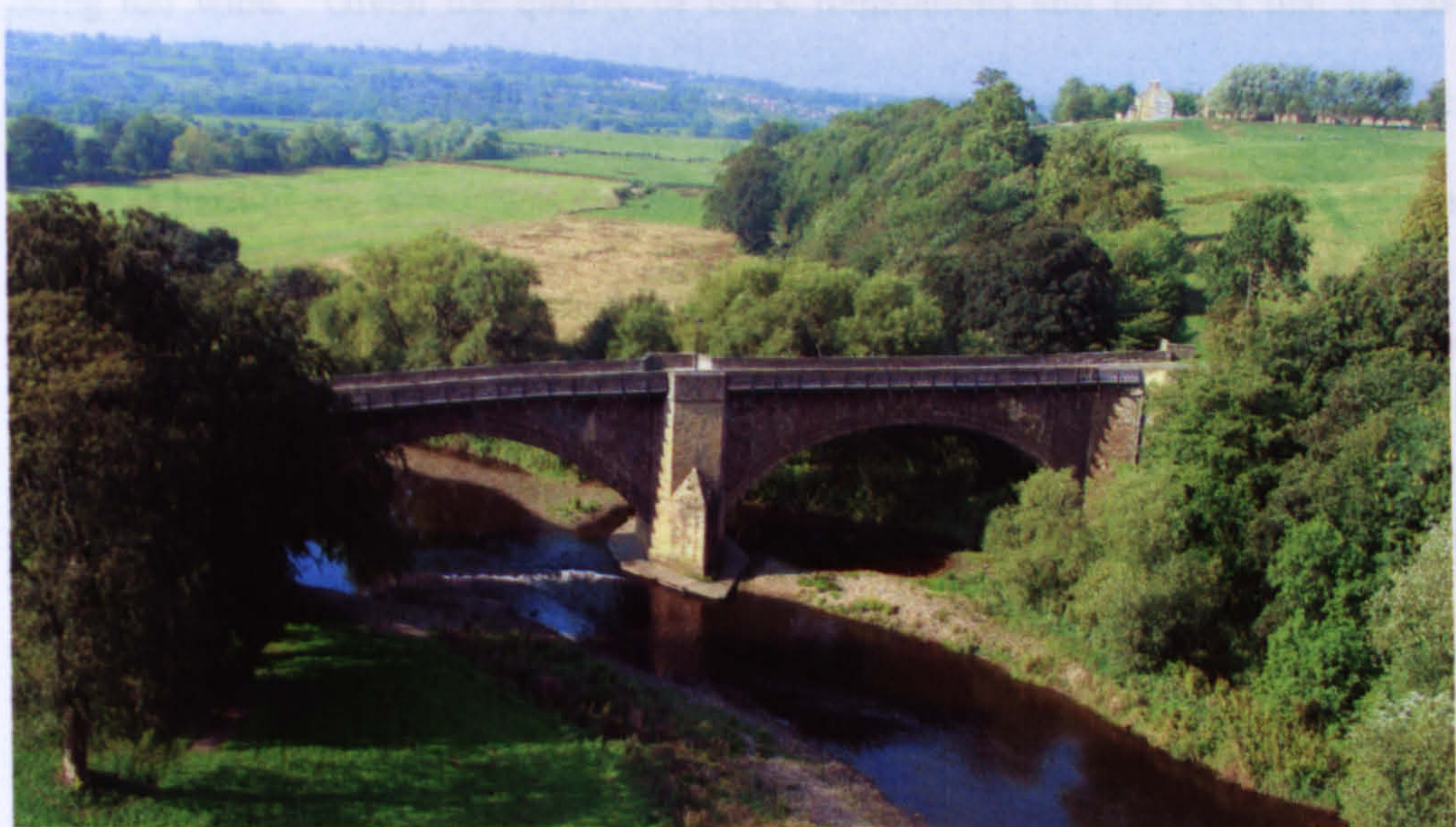
Figure 2-7 The 1388 bridge at Newton Cap, Bishop Auckland, Co. Durham
