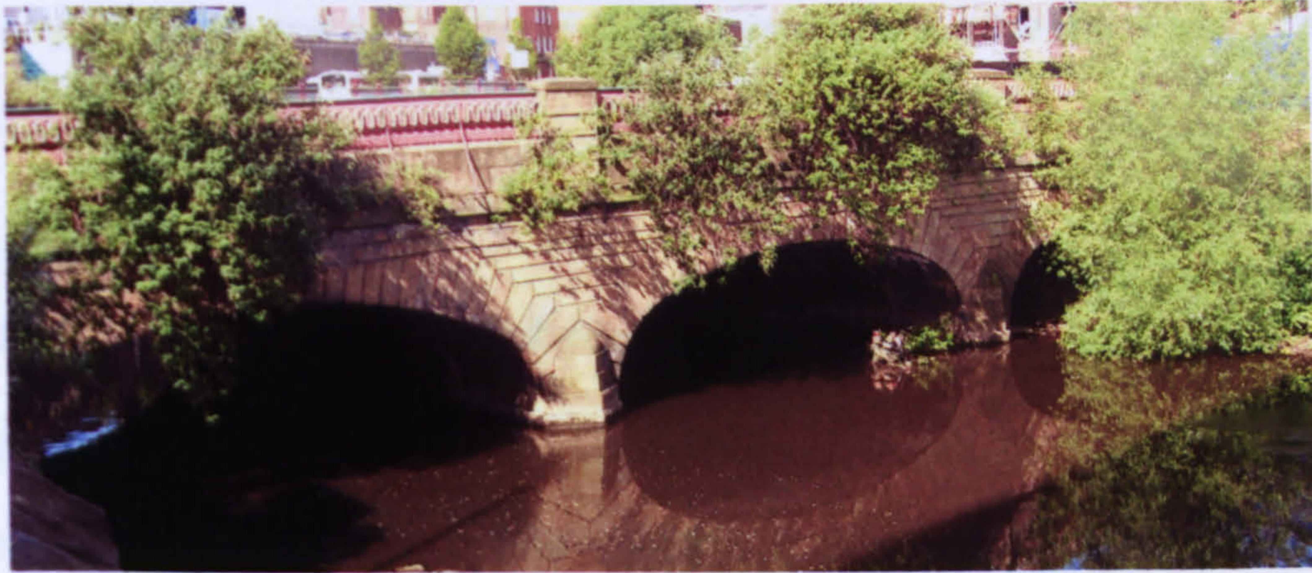
Figure 2-34 Blonk Street Bridge, Sheffield
