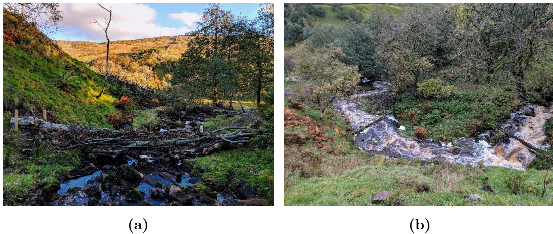
Figure 3.3: Photographs of (a) elevation and (b) plan view of typical leaky dams on the impact stream
