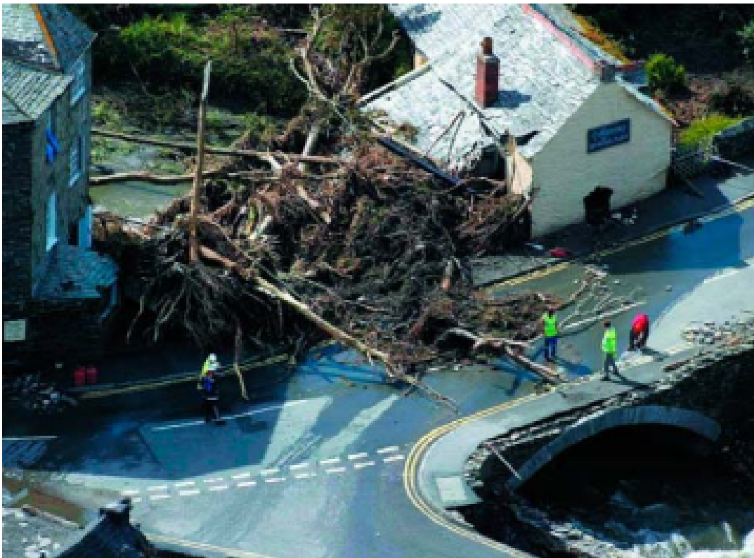
Figure 1.6: Woody debris blocking a bridge in Boscastle, Cornwall, during floods in 2004 ( Environment Agency, 2007b , p. 1)
