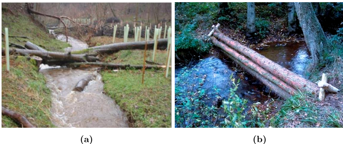
Figure 1.5: Examples of engineered leaky dams (a) A leaky dam in Belford, England which replicates natural wood accumulations, from Quinn et al. (2013, p.12) and (b) A uniform, engineered leaky dam in Pickering, England, from North York Moors National Park (2015)
