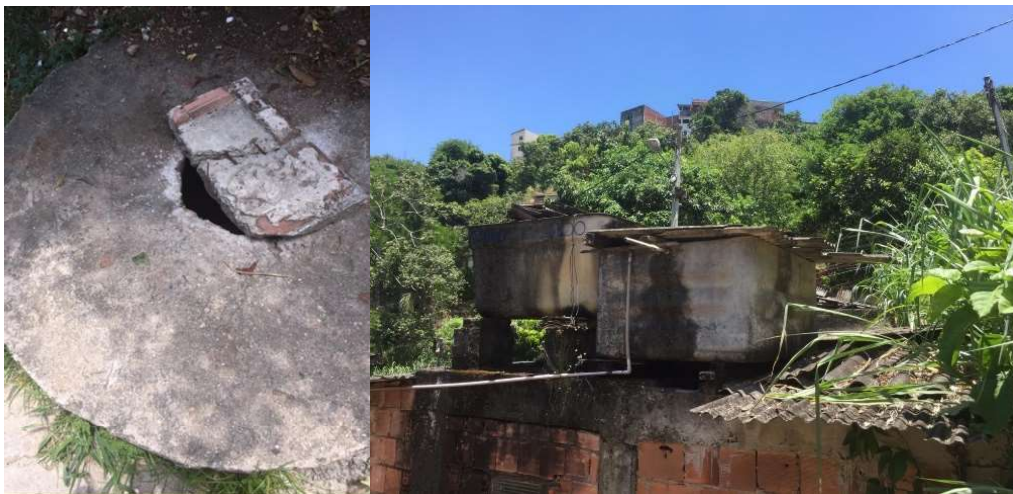
Figure 36 - Water tanks and cisterns found with openings and clean water inside. The biggest risk is not only contamination of it, and the entrance of small animals. But also if they are still, leads to mosquito's proliferation, that causes dengue fever outbreaks that are common to happen in summer in many different areas of the city but have a higher incidence in informal areas.
