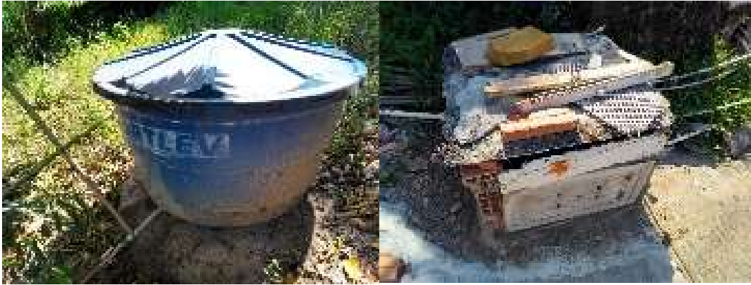
Figure 35 – Plastic water-tanks used by the majority of houses as their reservoirs. Old ones still use fibre ones. Plastic ones are preferred because of the better price, weight and ease of transportation. The second picture shows the hydro pump which belongs to the neighbour, and it fills his water-tank before reaching his. This dependency shifts a bit the water usage rates as he can't rely on having his reservoir filled up as he wishes. A water pipe network connects it, and its located on the bottom of the settlement pumping water from the formal network.
