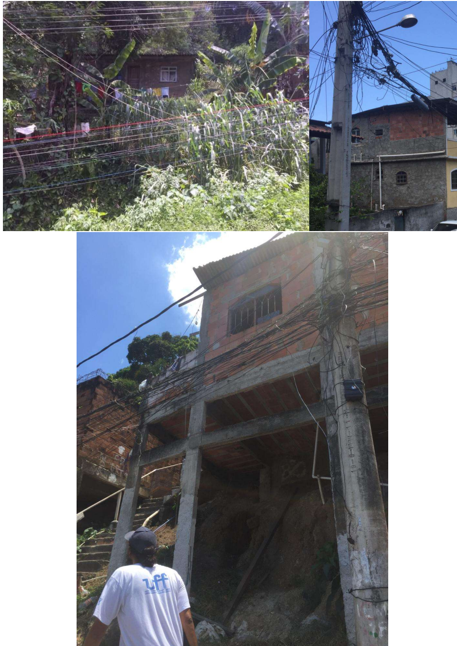
Figures 40a; b; 12 - The vast presence of informal illegal energy connections throughout the whole community.
