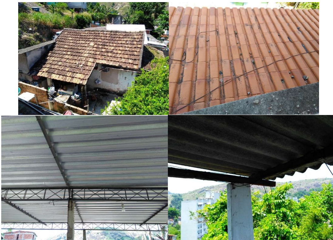
Figures 30 (a- d) – These older (a), newer (b) ceramic roof tiles and the zinc roof were seen on houses located side by side providing an element of heterogeneity. The fibrocement roof (d) as the cheapest option, is also apparently of common one on the dwellings.
