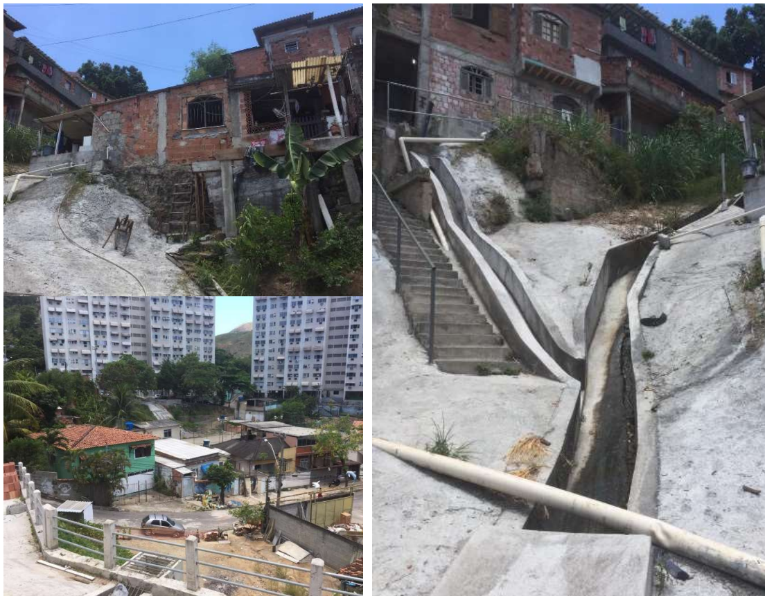
Figure 22 - Observe the hybridity of the formal infrastructure repairs done by the government after a landslide that killed 12 persons, merging directly into the informal houses. A couple of houses on an upper region are condemned and it was told to the researcher to still have residents in it.
