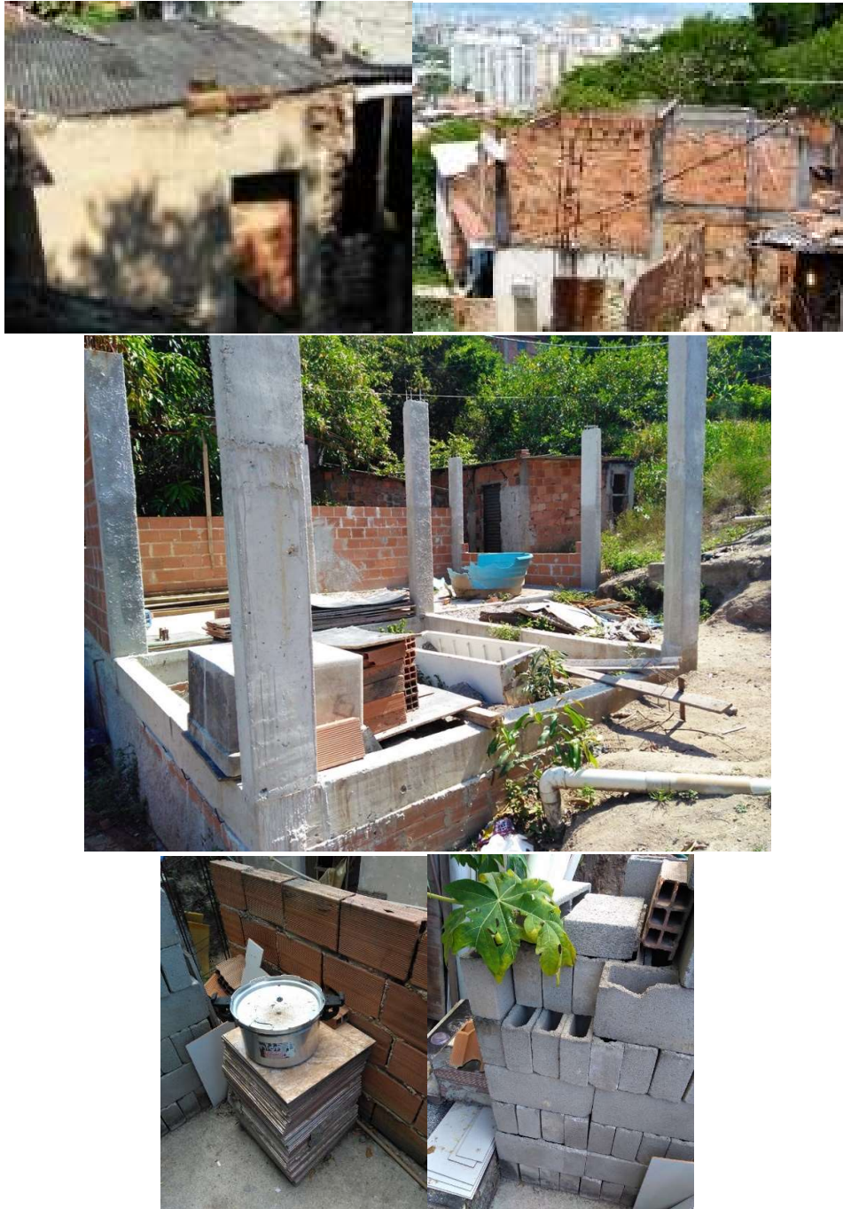
Figures 33 (a – i) – Dwellings under constructions, on several different stages. Unfinished houses with unstable or abandoned elements are very common. An indicative of different temporal processes is the construction materials that can be seen stored in many “courtyards” showing different shades of oxidation that can vary based on how long they are exposed to weathering when not stored under a roof.
