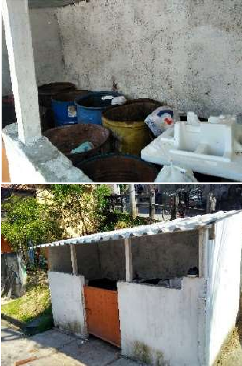
Figure 45 - Garbage depot. As reported, not large enough to attend the whole community. There is no separation of waste. It consists of 11 barrels of (guessing) 400-500 litres and it was constructed approximately 9 years ago by the local resident's association.
