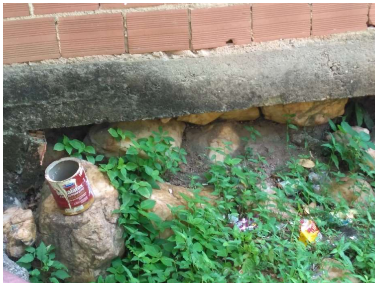
Figure 32 – The abundant rocks, apparently some sort of quartz, that occurs naturally in the hills of the community and are in this case sometimes seen in use. In this case, to sustain the foundation structure on some columns of this dwelling. It can also be observed the exposed pipe connections, water on the left, and sewage to the right connected to a junction box with the network.
