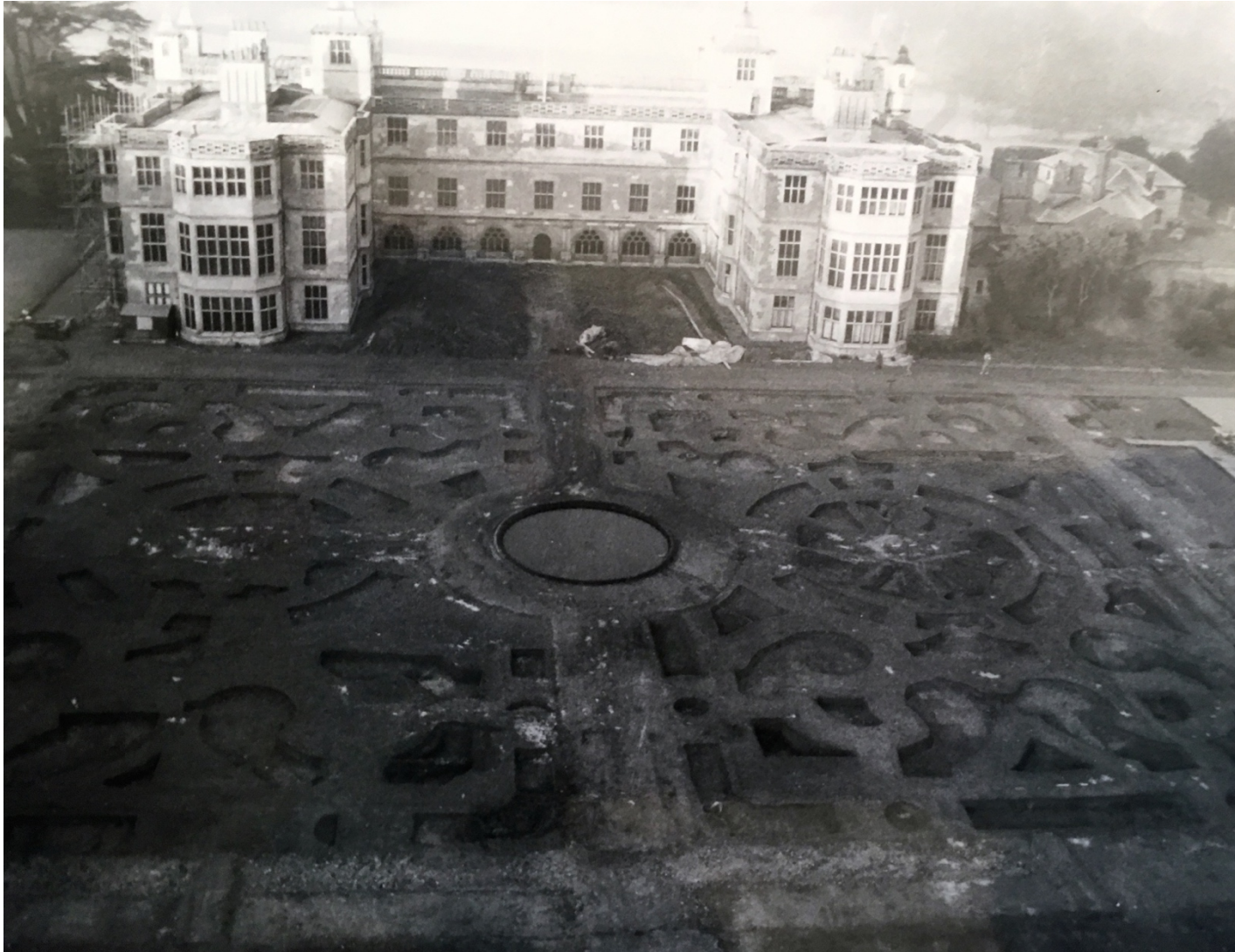
Figure 3.2: Photograph of the excavated main parterre area (site code JA) looking west. Taken by the Chelmsford Archaeological Trust, c.1986. © English Heritage.
